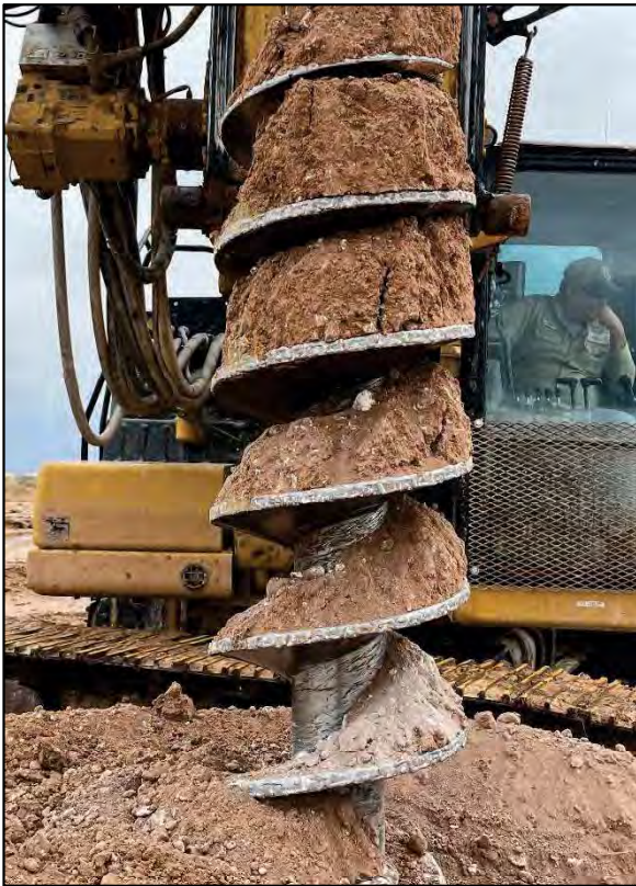
73-ft sample : auger (left), silt with limestone or dolomite (above)
