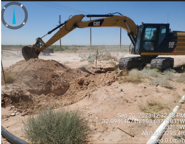
Photograph: 1 Date: 9/20/2023 Description: Excavation activities View: Southwest
