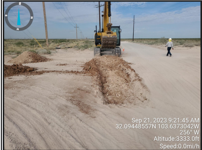
Photograph: 2 Date: 9/2/2023 Description: Excavation activities View: West
