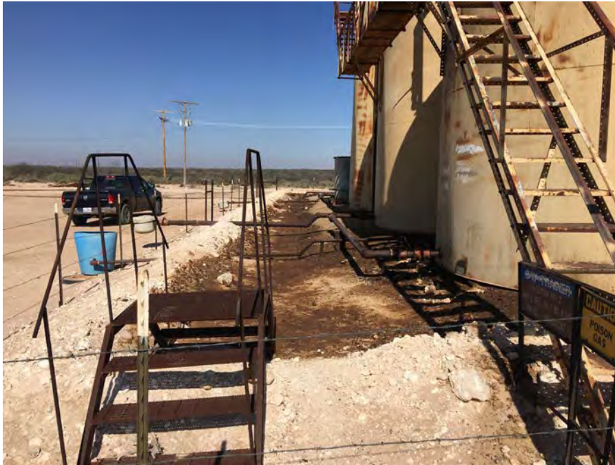
Figure 1: Southwest side of the tank battery showing the residual crude within the spill containment area. The fluids from the spill accumulated on this side of the containment and overflowed onto the location from the northwest side of the containment.
