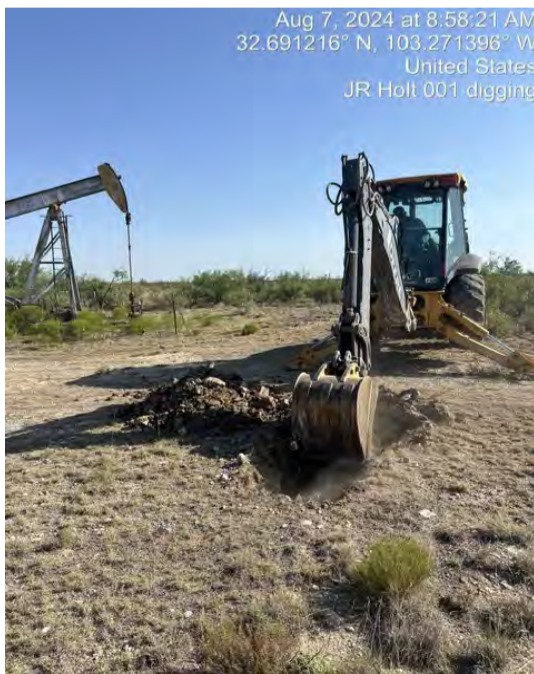
View to E of Sample 1 location (8/7/24).
