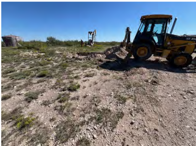
View to E of excavating (9/25/24).
