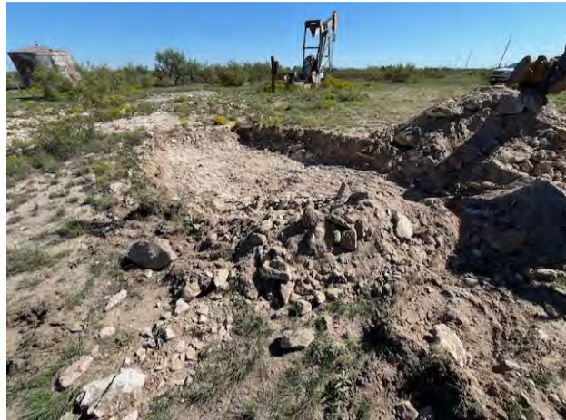
View to NE of excavation (9/25/24).
