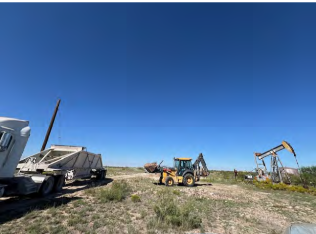
View to W of loading dump truck with excavated soil (9/25/24).
