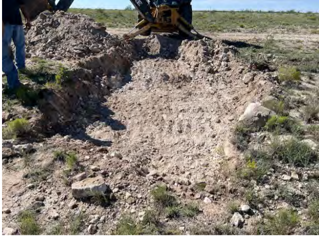
View to S of excavation (9/25/24).
