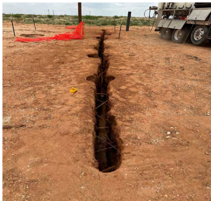
Hydro-vac to expose lines
