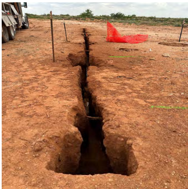
Hydro-vac to expose lines
