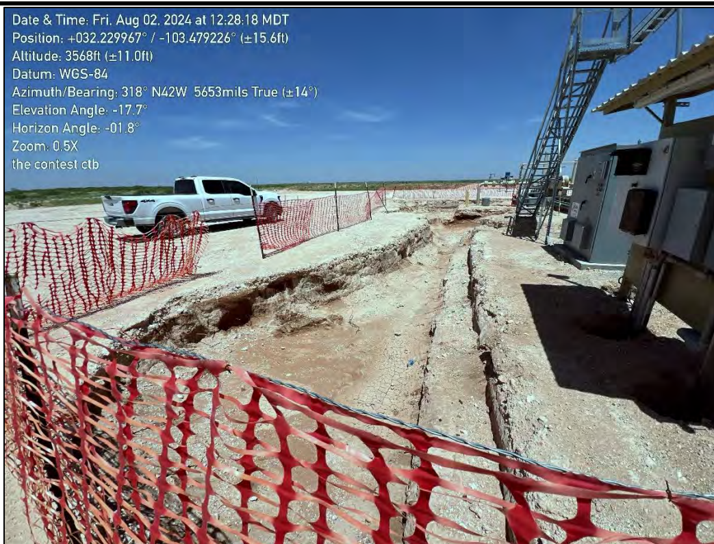
PHOTO 4: Northwest view of excavation extent. 8/02/2024
