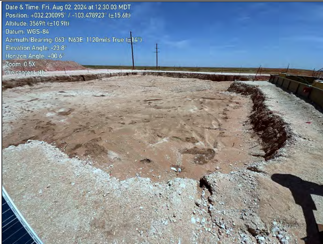
PHOTO 3: Northeast view of excavation extent. 8/02/2024
