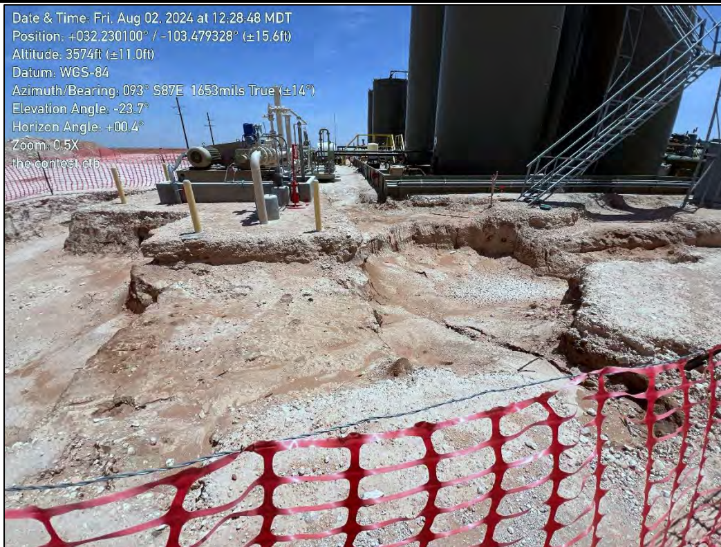
PHOTO 5: Southeast view of excavation extent. 8/02/2024
