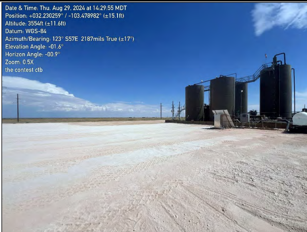
PHOTO 10: Southeast view during Site restoration activities. 8/29/2024
