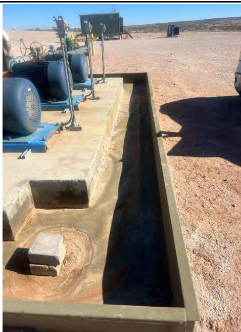
Photograph 3 Date: 01/13/2023 Description: Liner inspection activities. View: East
