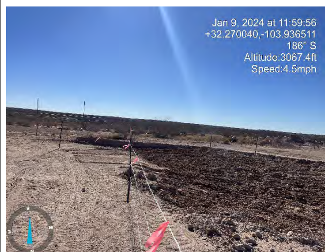
Photograph 3 Date: 01/09/2024 Description: Excavation activities View: South
