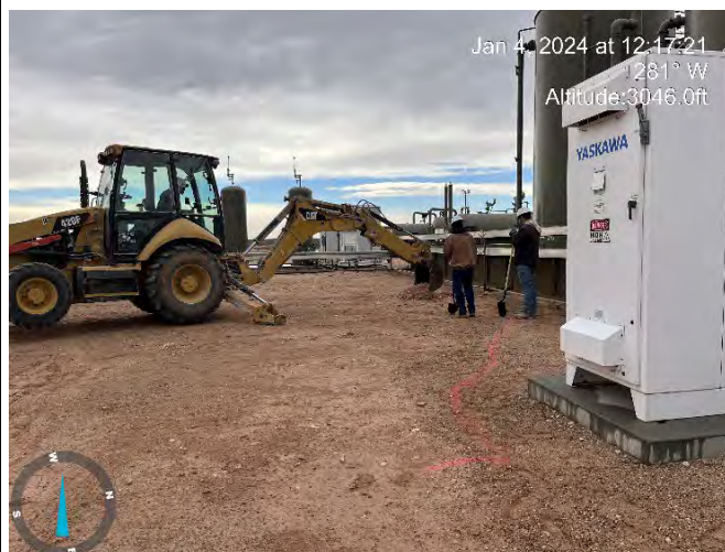
Photograph 1 Date: 01/04/2024 Description: Starting excavation activities View: West
