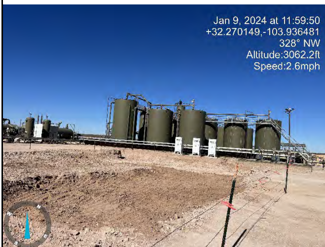
Photograph 2 Date: 01/09/2024 Description: Excavation activities View: Northwest
