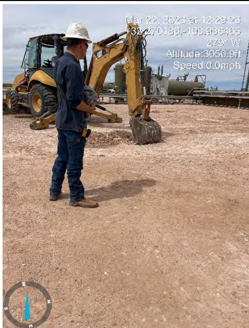
Photograph 3 Date: 3/22/2023 Description: Delineation activities, area of PH03 View: West
