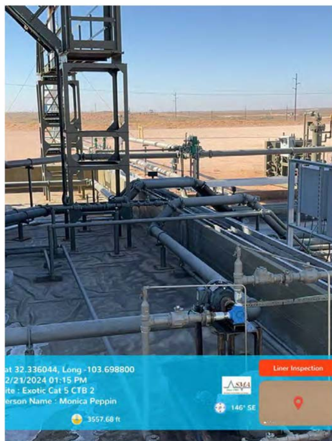
Photograph #4: liner in tank containment from east side
