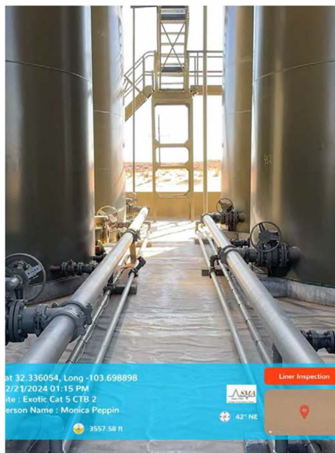
Photograph #5: Liner between tanks
