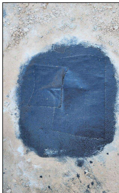
Photograph: 12 Date: 11/20/2024 Description: BH01 patched. View: N/A
