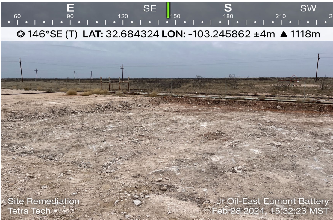
View of Remediation Activities – View Southeast
