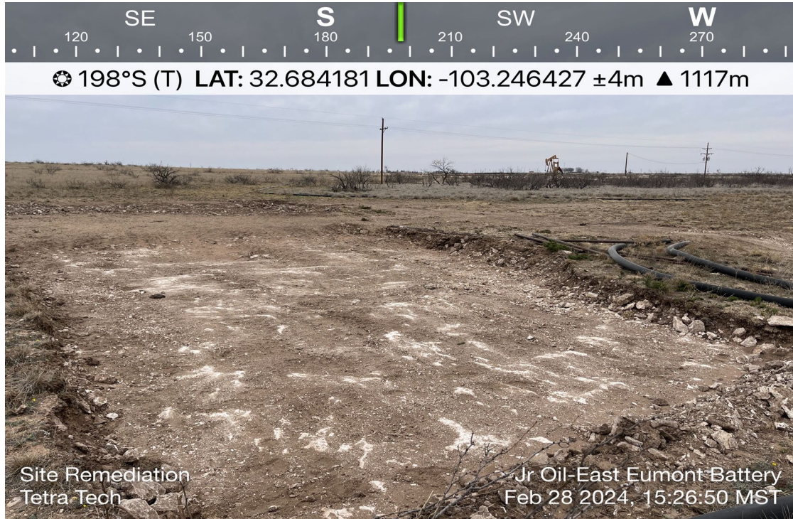
View of Remediation Activities – View South
