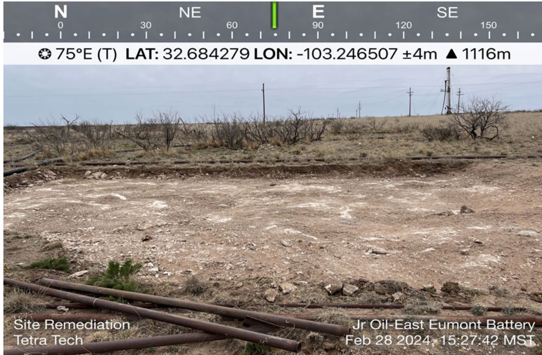
View of Remediation Activities – View Northeast
