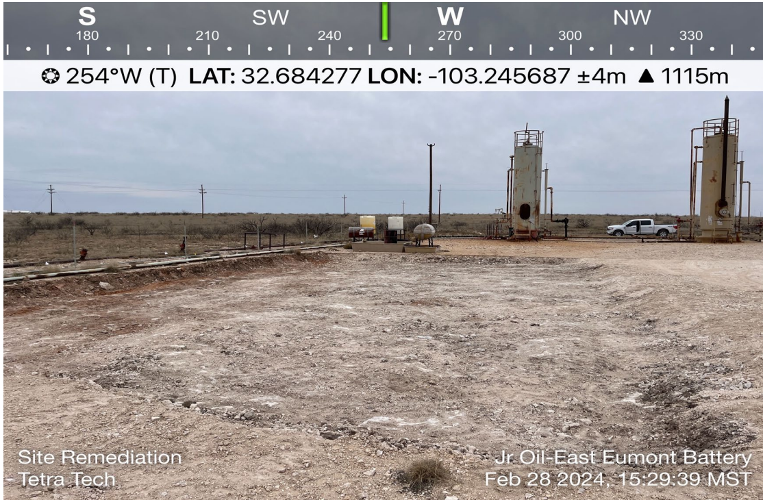
View of Remediation Activities – View West
