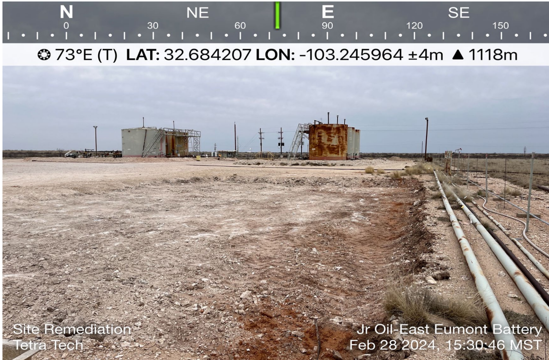
View of Remediation Activities – View Northeast
