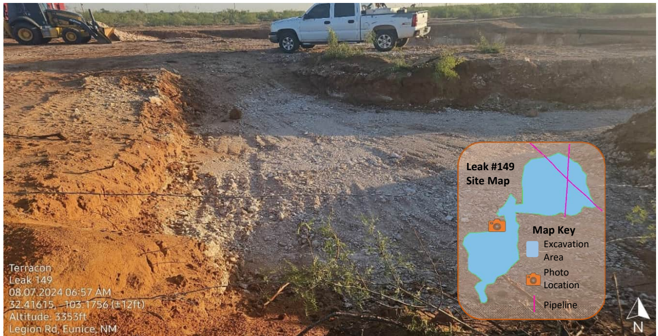
Photo 13 Excavation complete southeast of pipeline intersection 4' bgs looking north
