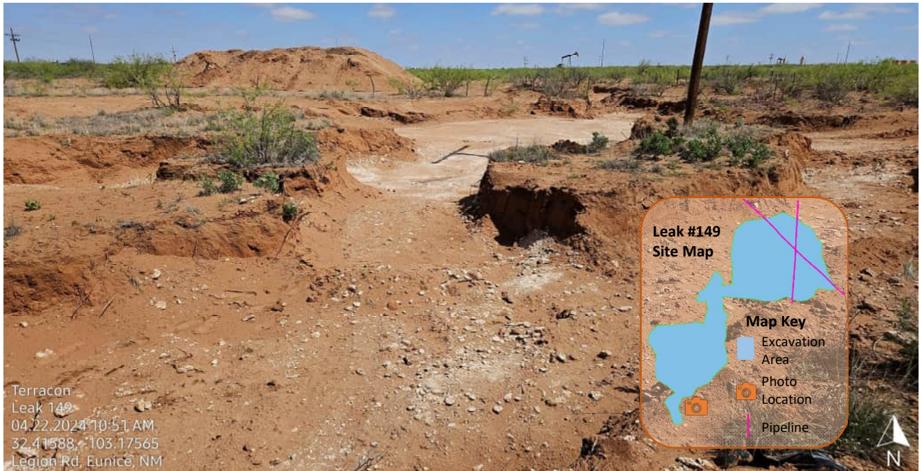
Photo 15 Excavation in progress around powerline / Southern Area looking north
