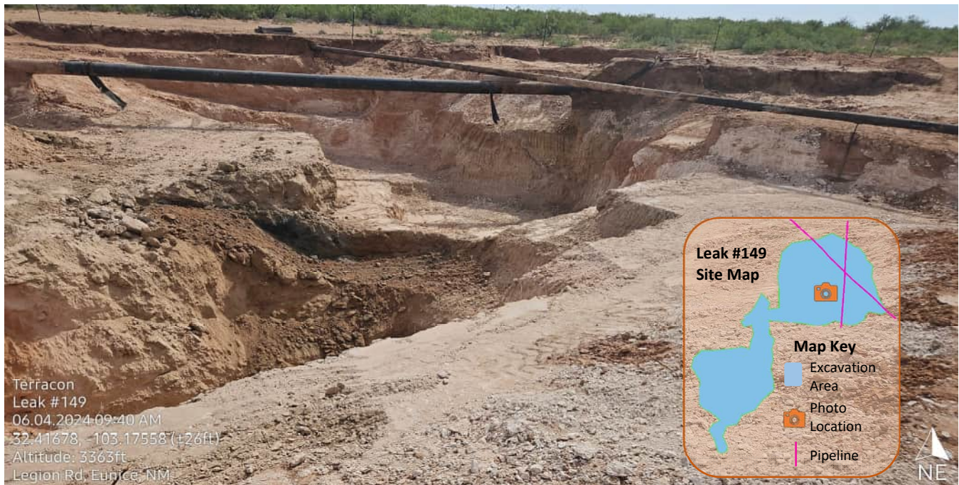
Photo 7 View of excavation in progress staining at 12' bgs looking northeast
