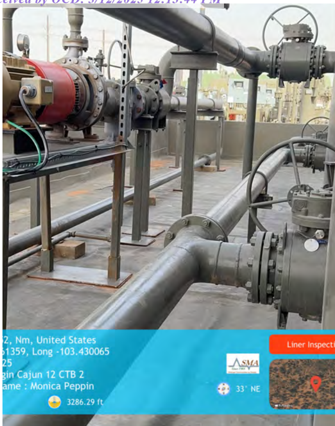
Photograph #11: Northwest area of containment.
