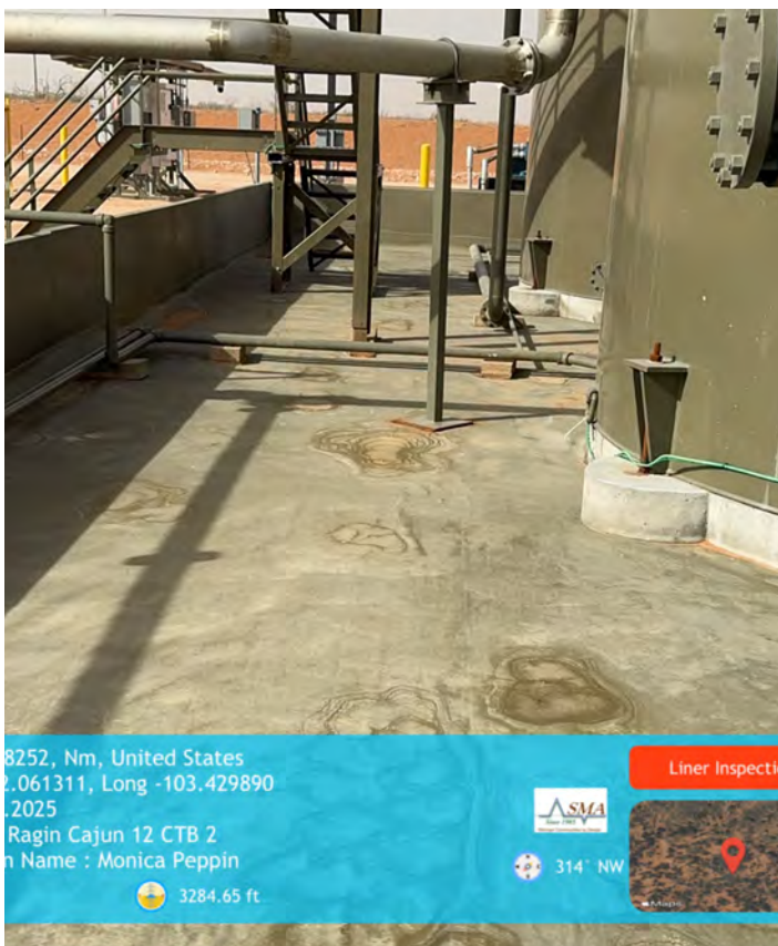
Photograph #7: Facing west from northeast corner.
