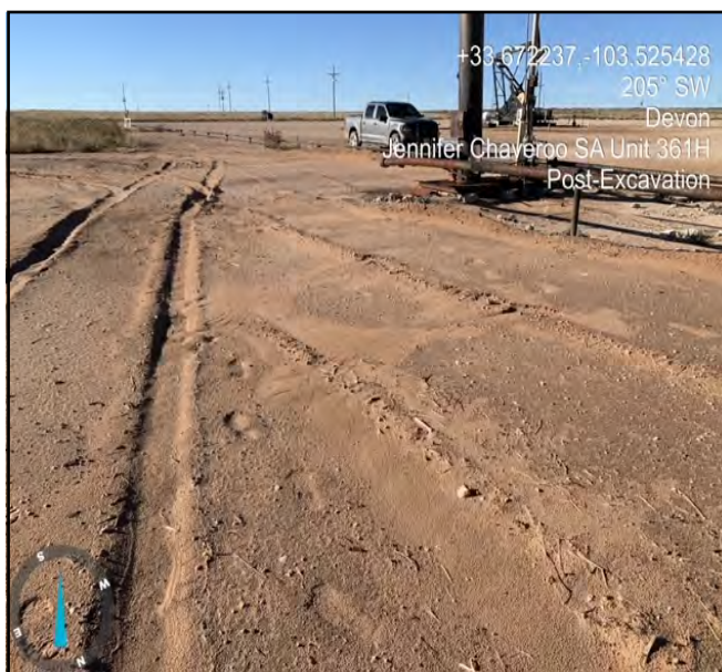
Photograph of the excavation backfilled with clean material facing Southwest.
