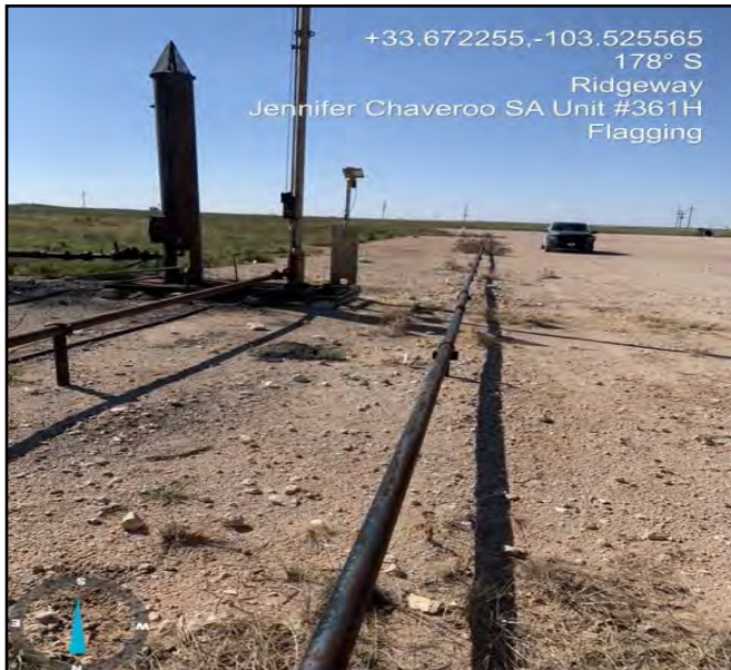
Photo of site being flagged for excavation facing South.
