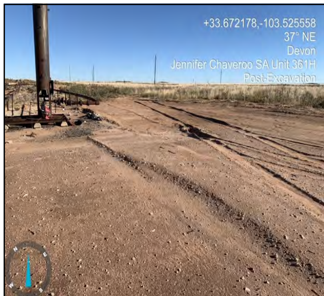
Photograph of the excavation backfilled with clean material facing Northeast.
