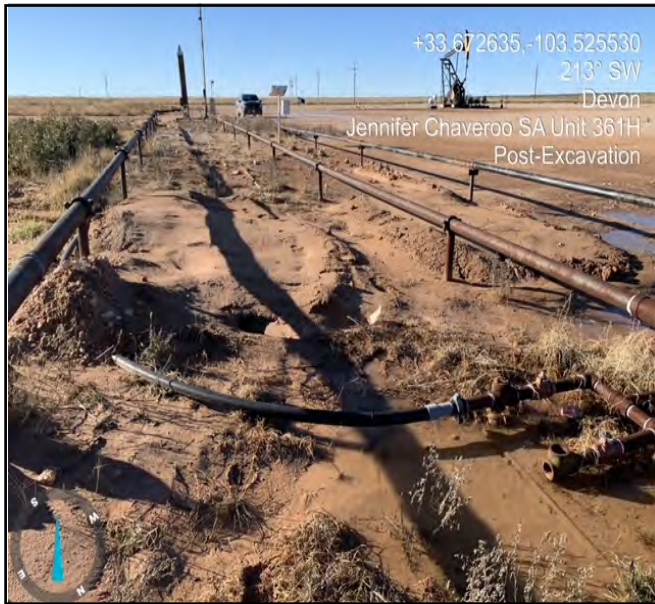
Photograph of the excavation backfilled with clean material facing Southwest.
