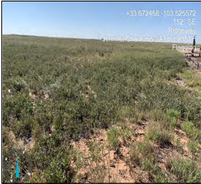
Photo of site being flagged for excavation facing Southeast.
