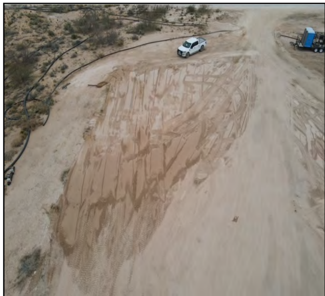
Photo of the excavation site completely backfilled with clean material. Taken by a drone.
