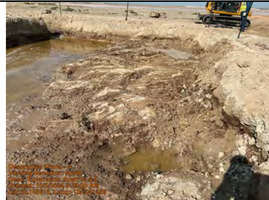
Excavation down to 4.5'
