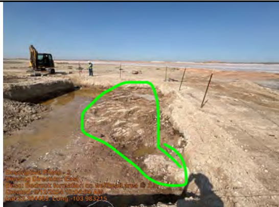
Bedrock formation on wellhead area @ 2.5'
