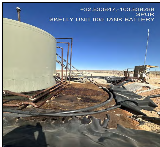
Photo of compromised area located on the east side of the lined containment.
