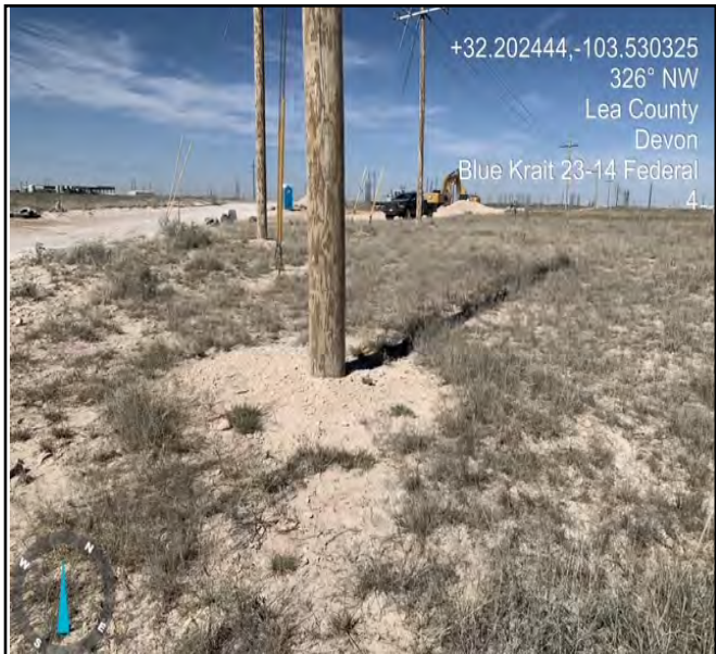
Point of reference area 4, Facing Northeast.
