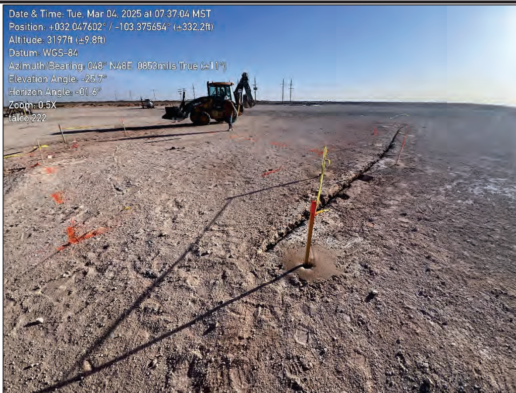
PHOTO 4: Northeastern view during preparation for excavation activities. 3/4/2025
