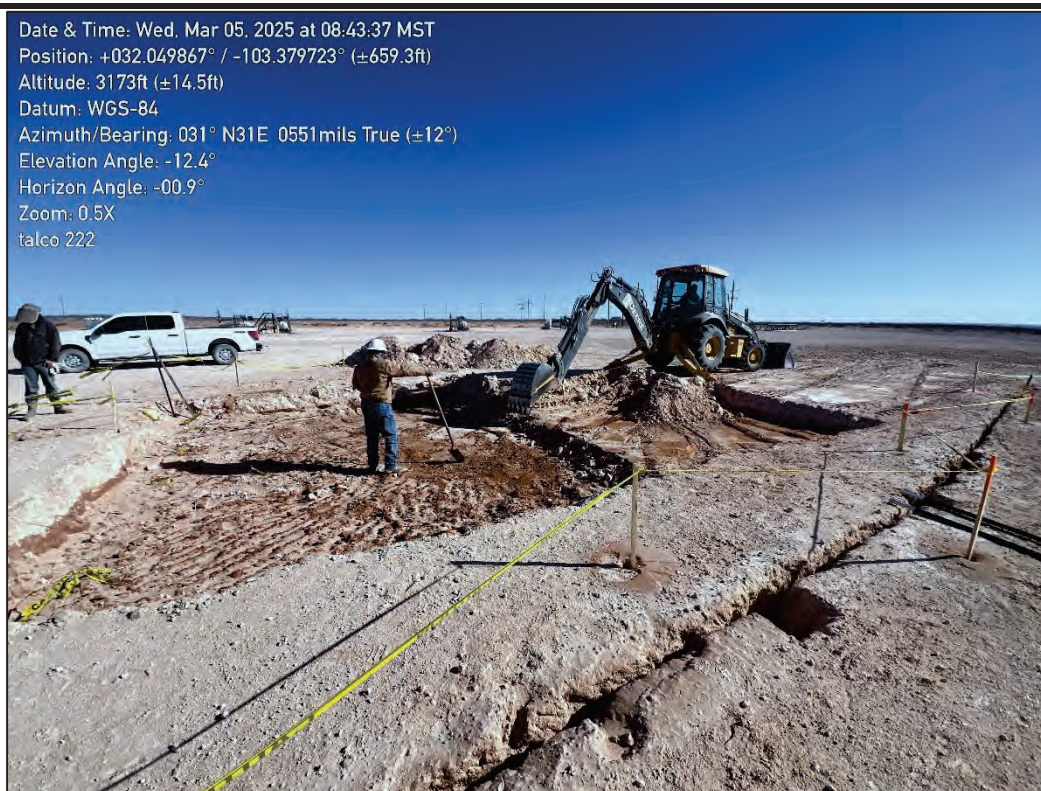
PHOTO 6: Northeastern view during excavation activities. 3/5/2025
