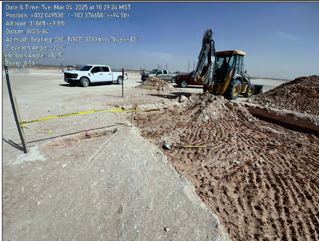
PHOTO 5: Northeastern view during excavation activities. 3/4/2025
