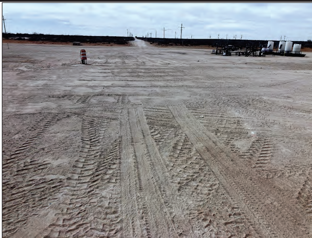
PHOTO 8: Northwestern view following restoration activities. 3/17/2025
