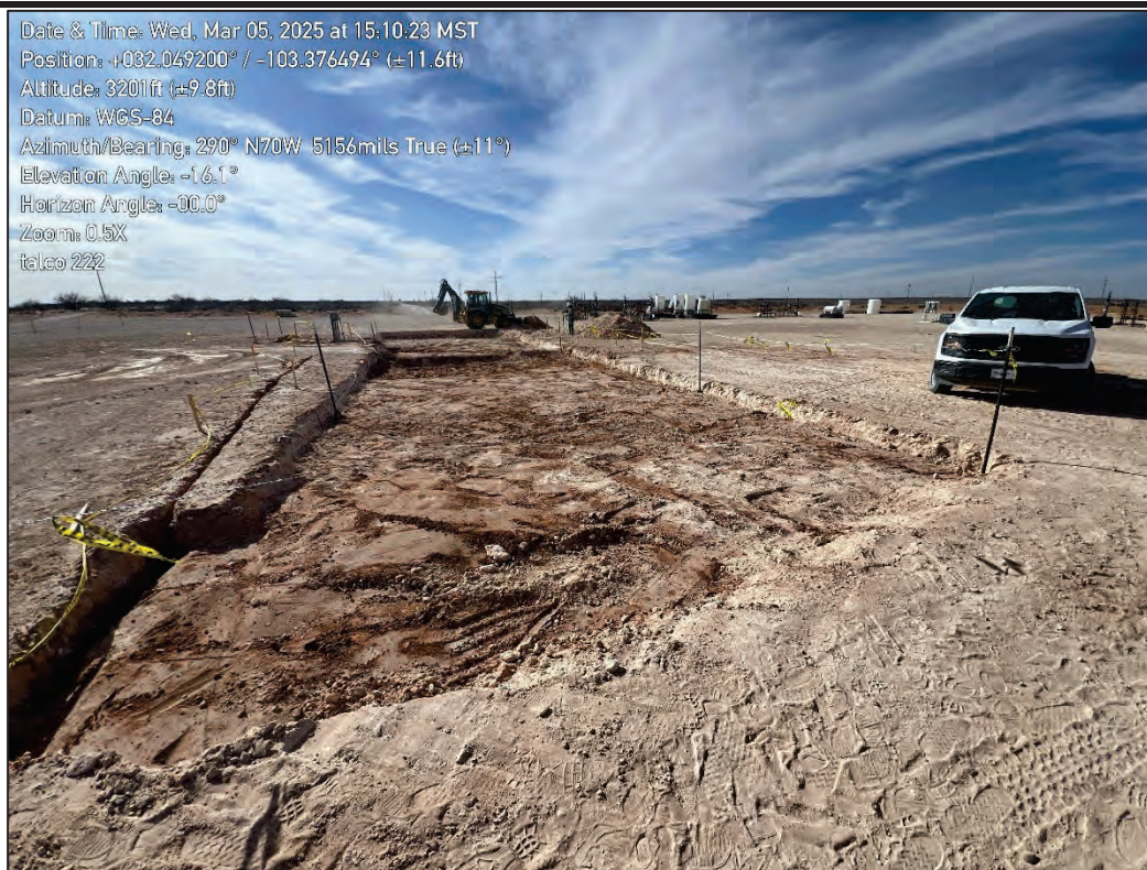
PHOTO 7: Northwestern view of excavation extent. 3/5/2025
