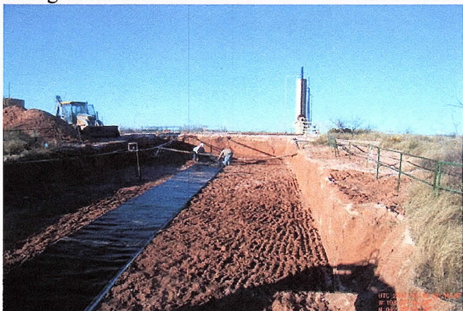
Installing 20-mil, reinforced liner at 4.5 ft bgs, facing north
