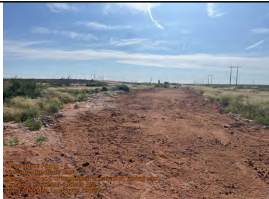
West end of backfilled excavation facing east.
