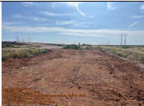
Mid point of backfilled excavation facing east.
