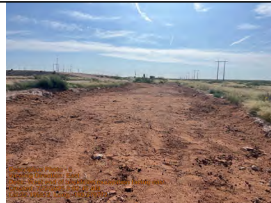
West end of backfilled excavation facing east.
