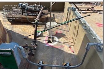
Photograph: 9 Date: 8/22/2025 Description: Liner Inspection Activites; tear located
