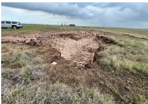
View to N of excavation (6/24/25).
