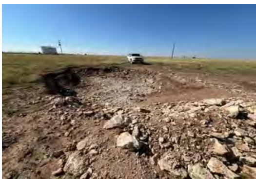
View to SE of excavation (8/22/25).
