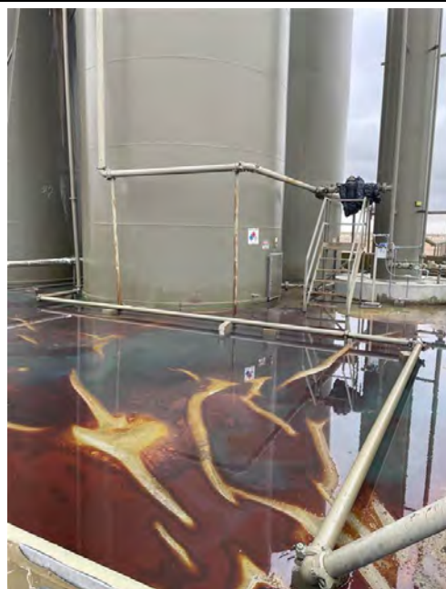
Photograph 4 Description: Spill area (nAPP2517723595) View: East Date: 6/25/25
