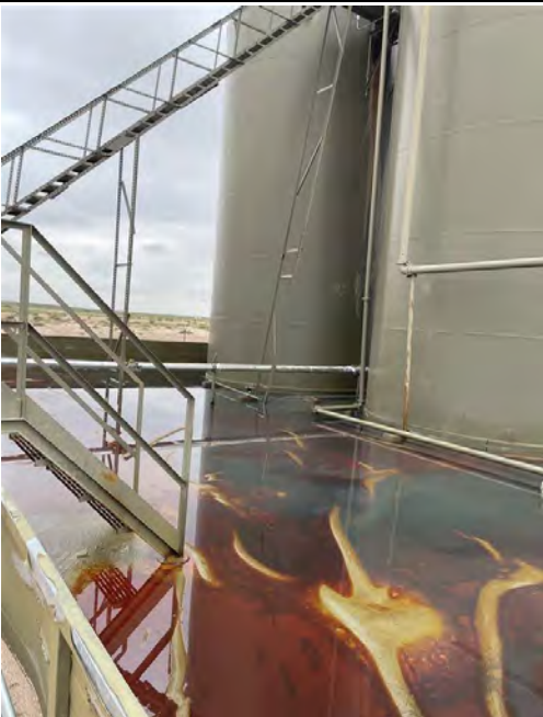
Photograph 3 Description: Spill area (nAPP2517723595) View: Northeast Date: 6/25/25
