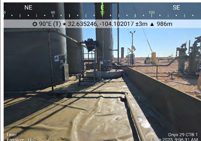
Photograph 12 Description: Liner Inspection View: East
