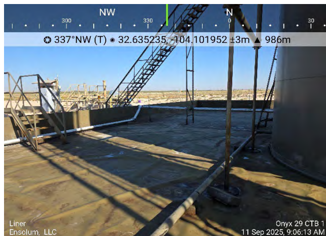
Photograph 11 Description: Liner Inspection View: Northwest
