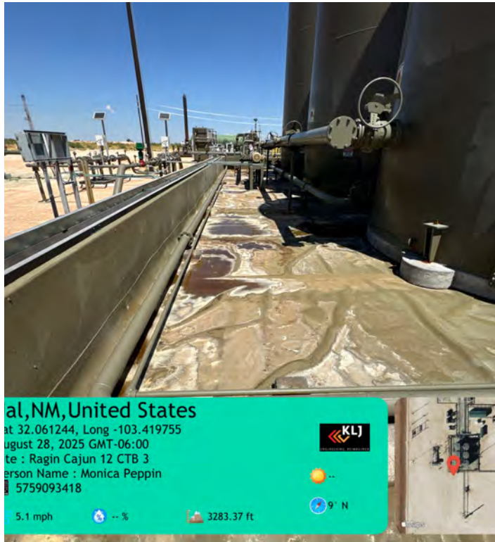
Facing north from southwest corner.
