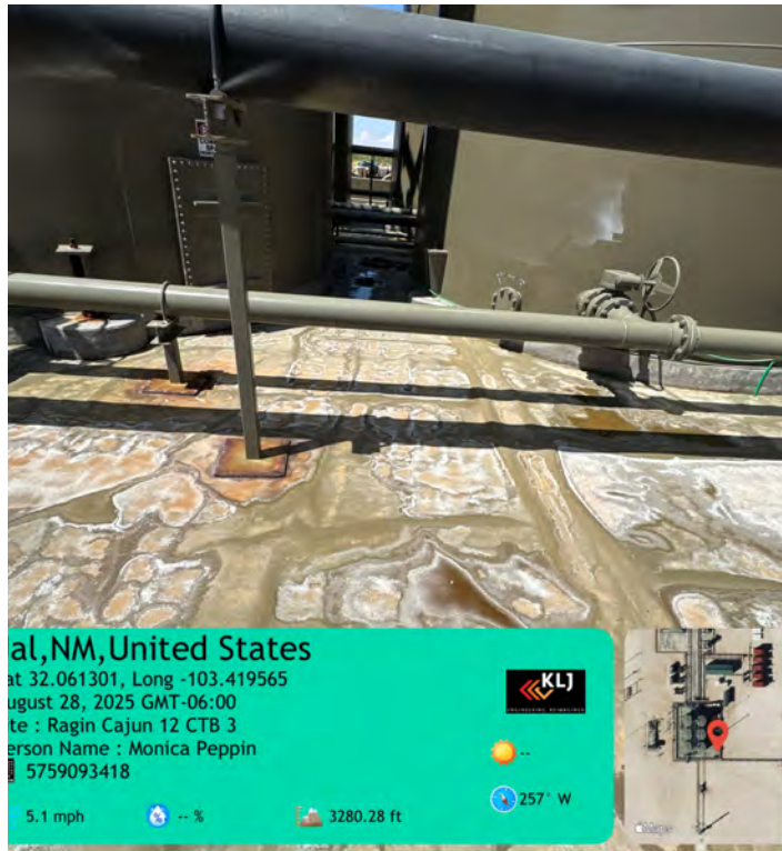
Liner between tanks facing west middle section.
