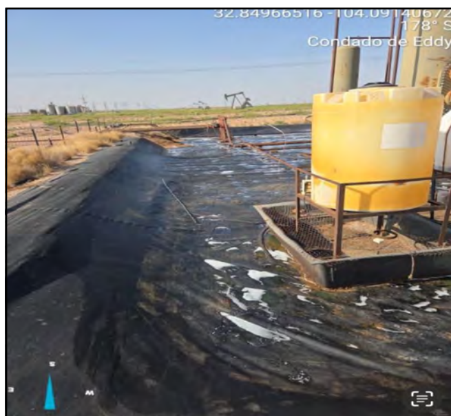
Photo of liner inspection post power wash facing south.
