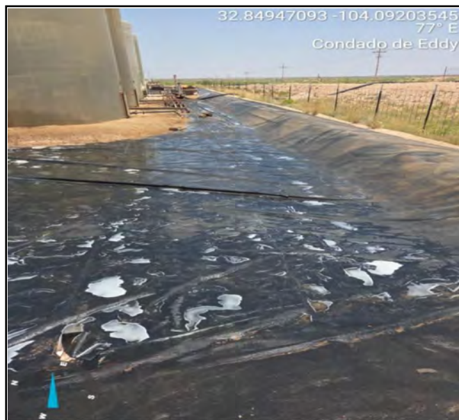
Photo of liner inspection post power wash facing east.
