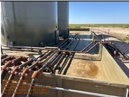
Northwest corner facing south
