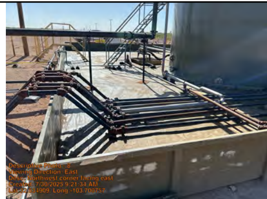
Northwest corner facing east
