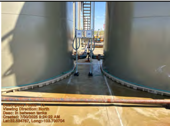
In between tanks
