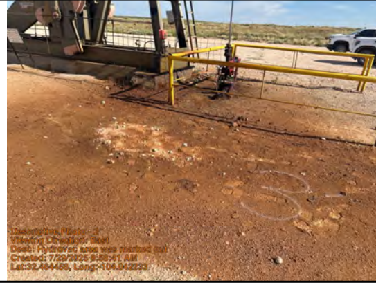
Hydrovac area was marked out
