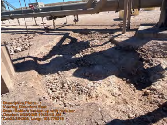
Boulders broken up with rock bar
