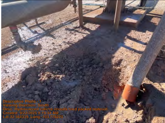
Hydrovaccated caliche reveals hard packed material
