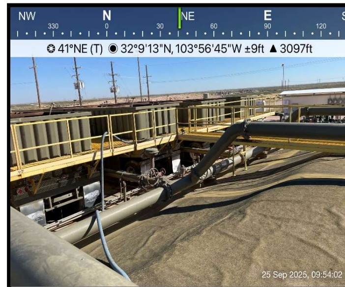
View of secondary containment
