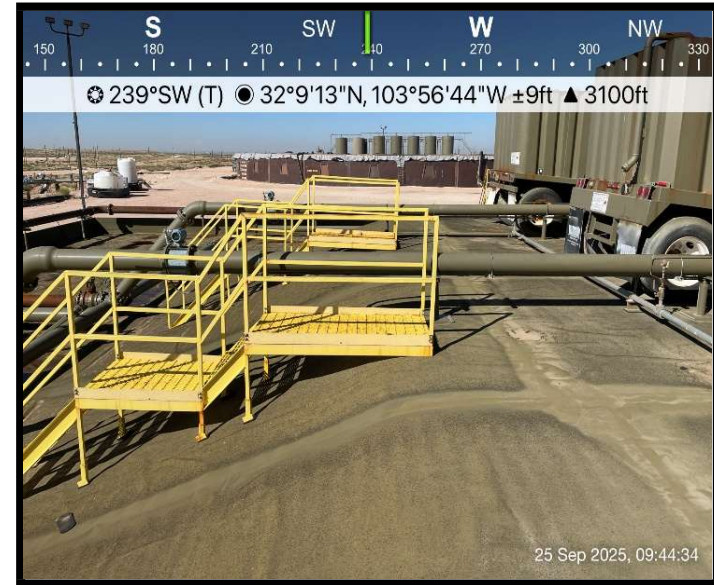
View of secondary containment
