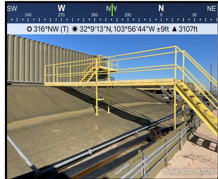
View of secondary containment
