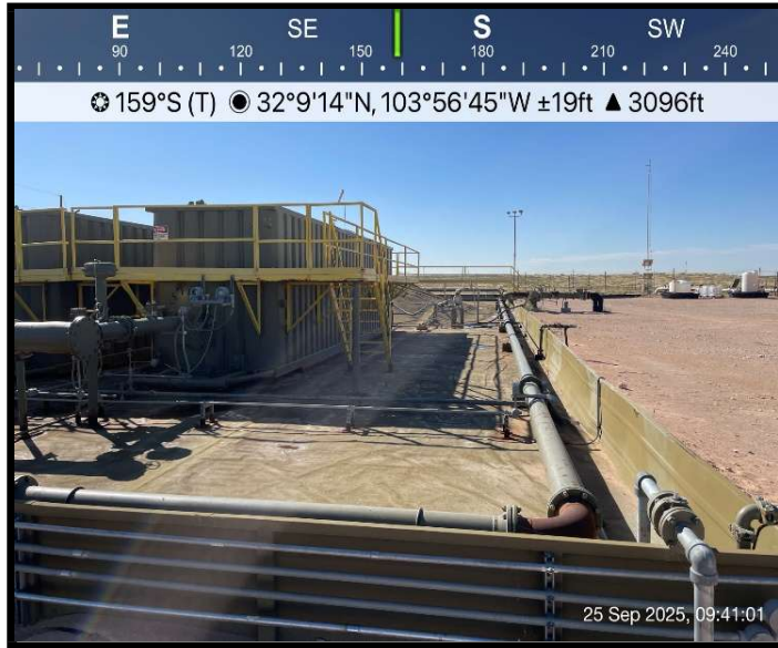
View of secondary containment
