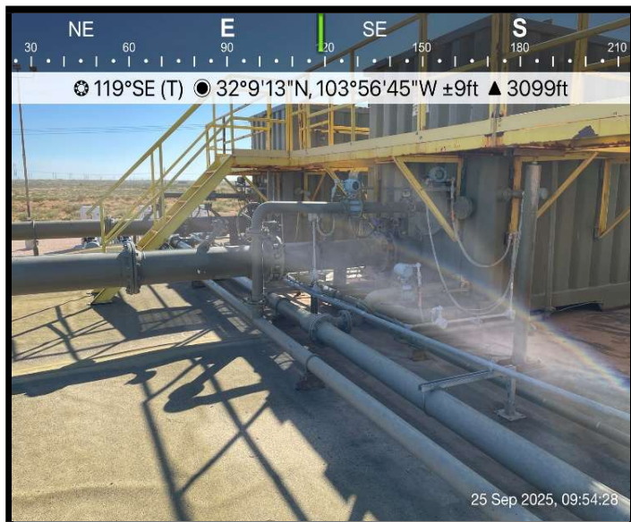
View of secondary containment
