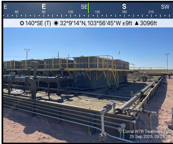
View of secondary containment
