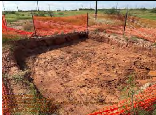
Northwest corner of excavation to 2' bgs facing southeast.
