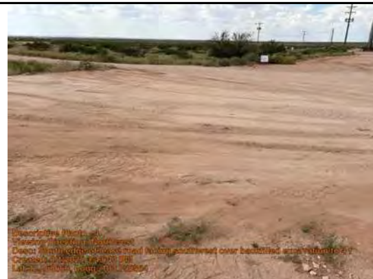
South edge of lease road facing southwest over backfilled excavation to 4 feet bgs.
