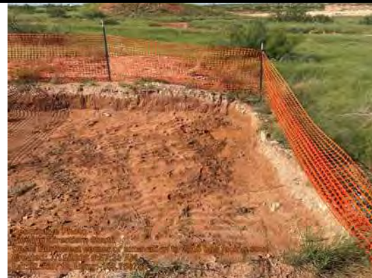
Northwest corner of excavation to 2' bgs facing south.
