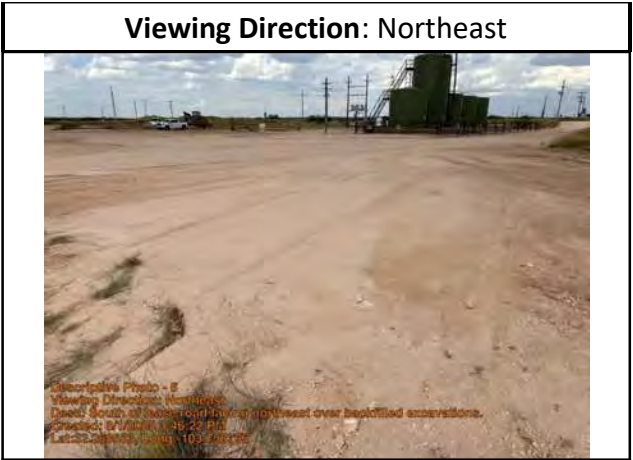
South of lease road facing northeast over backfilled excavations.
