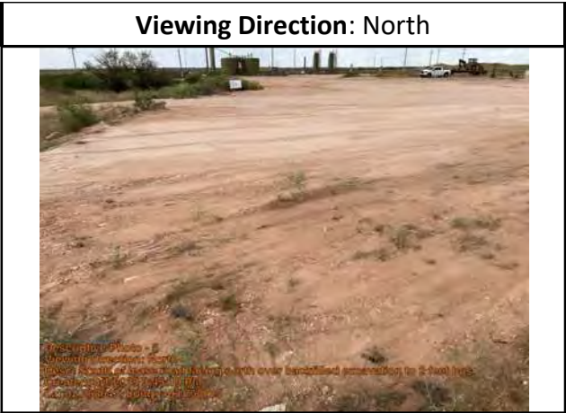
South of lease road facing north over backfilled excavation to 2 feet bgs.
