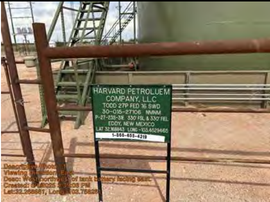
West-northwest of tank battery facing east.
