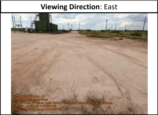
South of lease road facing east over backfilled excavations.
