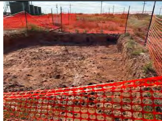
Southwest corner of excavation to 2' bgs facing east.
