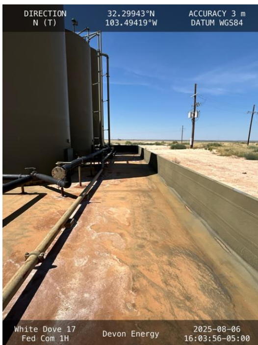
Photo 7 View of eastern portion of containment facing north.
