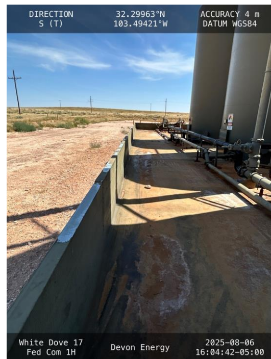
Photo 8 View of eastern portion of containment facing south.
