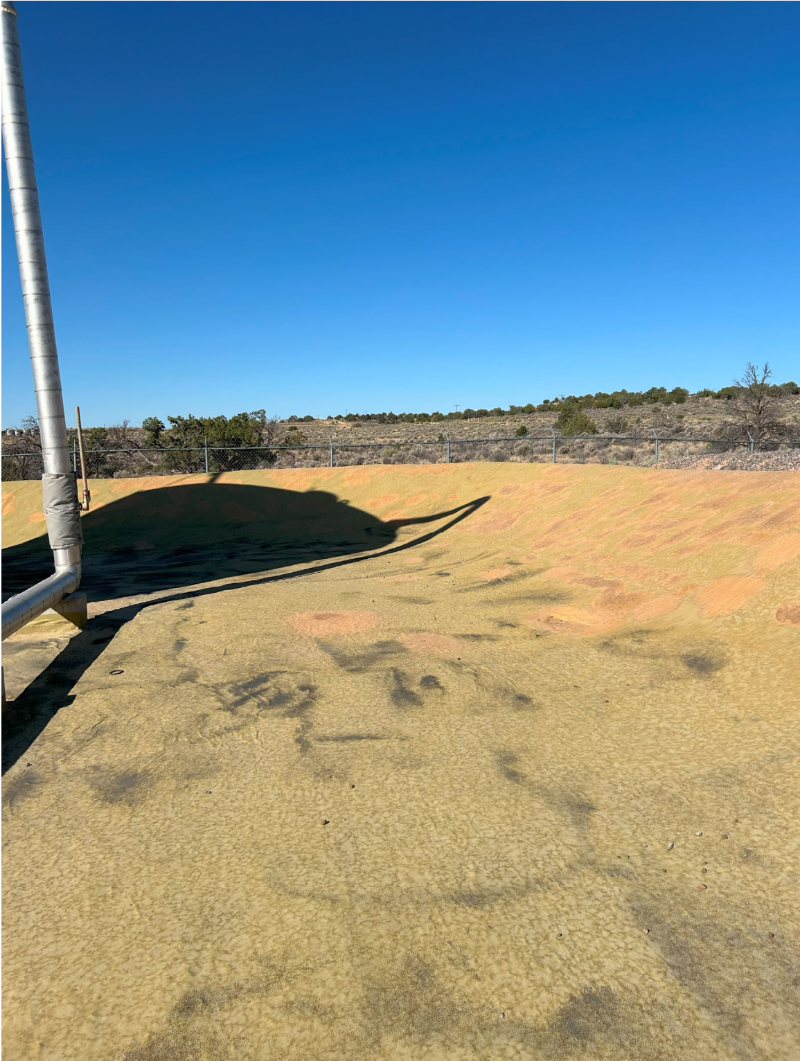
Photo 3: View of the secondary containment system.
