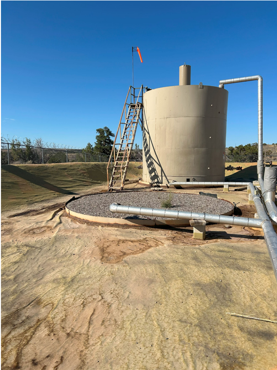
Photo 4: View of the secondary containment system.
