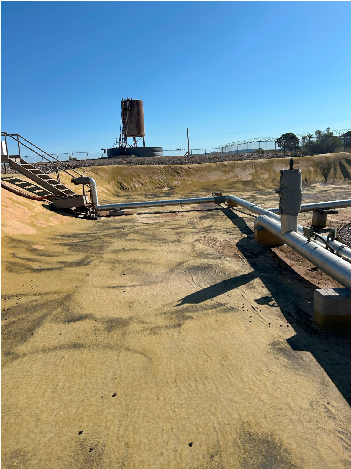
Photo 2: View of the secondary containment system.
