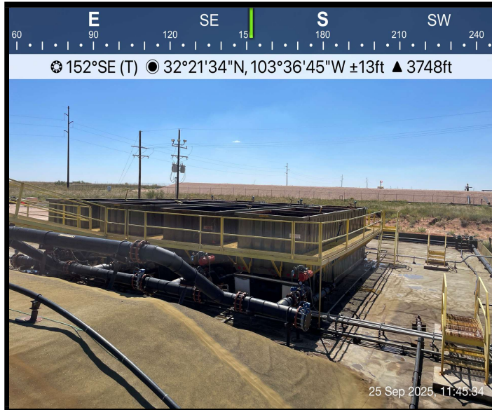
View of secondary containment
