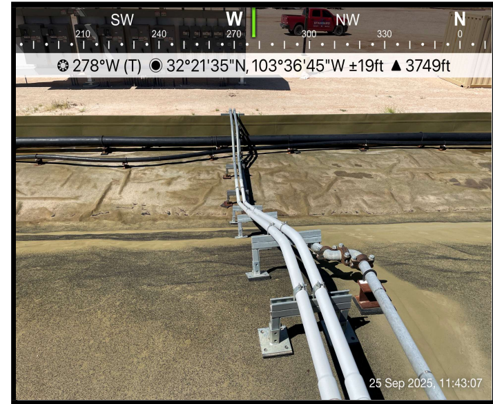
View of secondary containment
