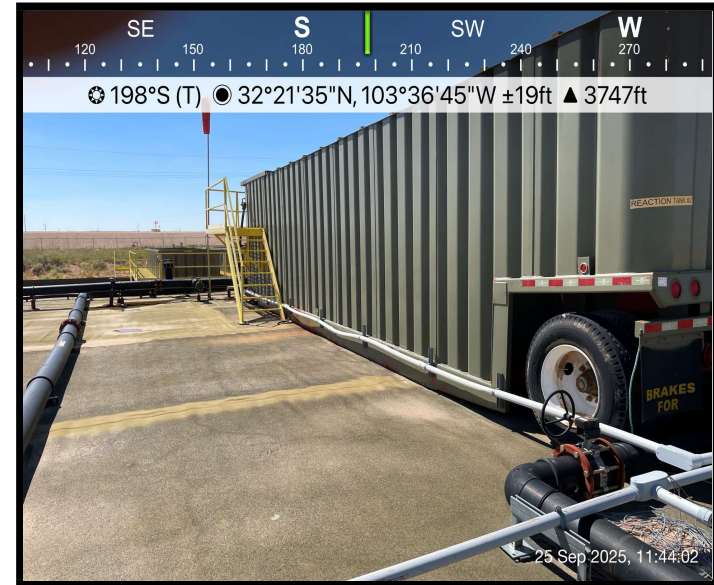
View of secondary containment
