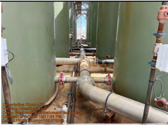
West end of containment facing east.
