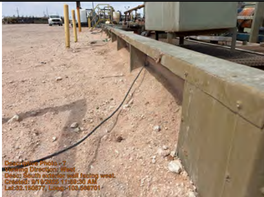
South exterior wall facing west.
