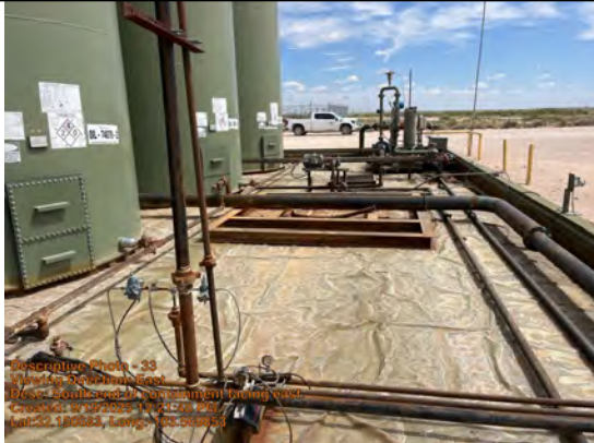
South end of containment facing east.
