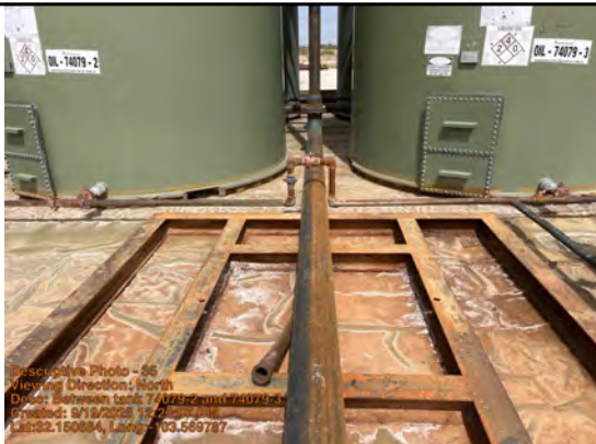
Between tank 74079-2 and 74079-3.
