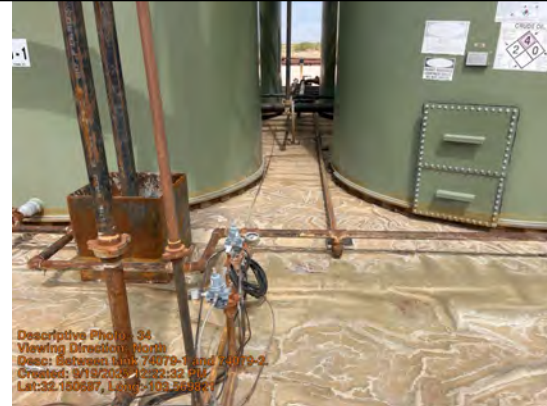
Between tank 74079-1 and 74079-2.
