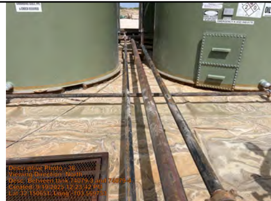
Between tank 74079-3 and 74079-4.
