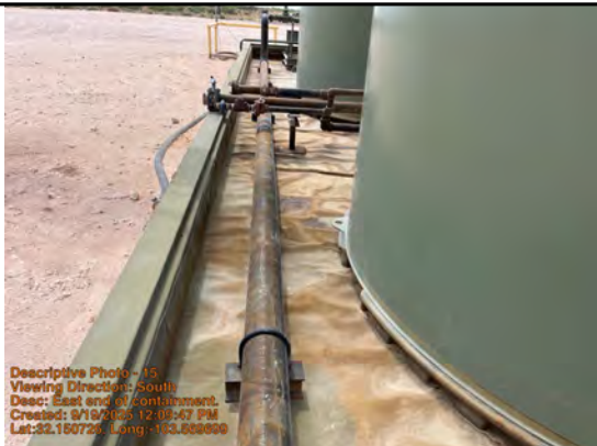
East end of containment facing south.
