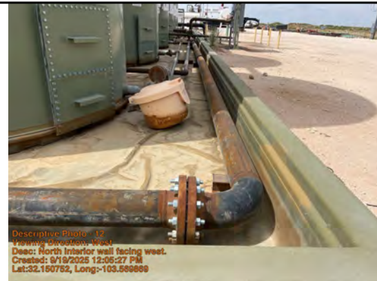
North interior wall facing west.
