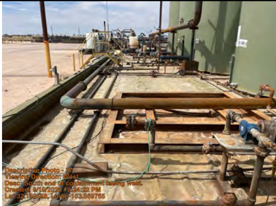
South end of containment facing west.
