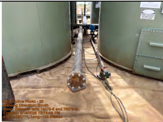
Between tank 74079-8 and 74079-W3
