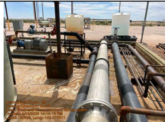
West end of containment facing south.
