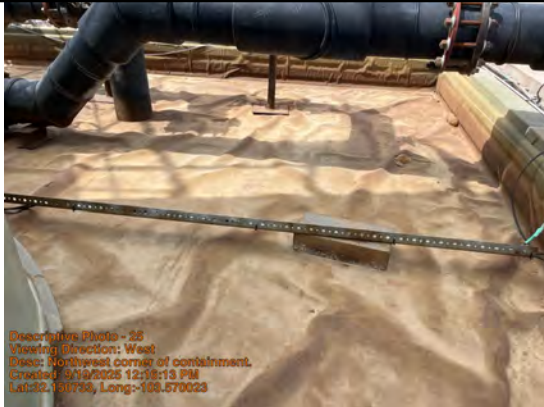
Northwest corner of containment.
