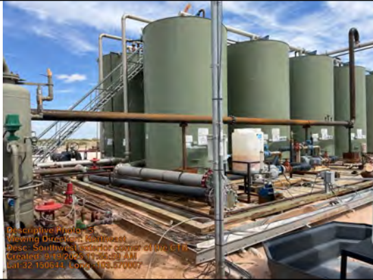
Southwest exterior corner of the CTB.
