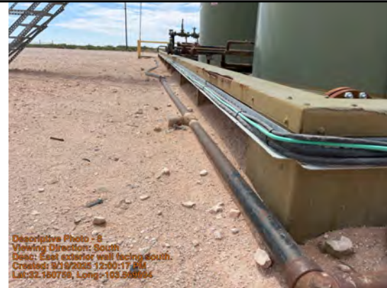
East exterior wall facing south.
