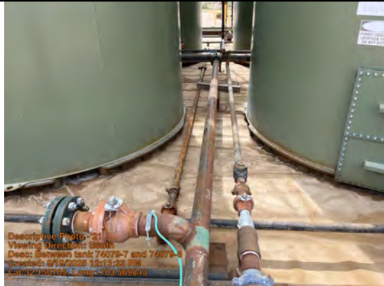
Between tank 74079-7 and 74079-8
