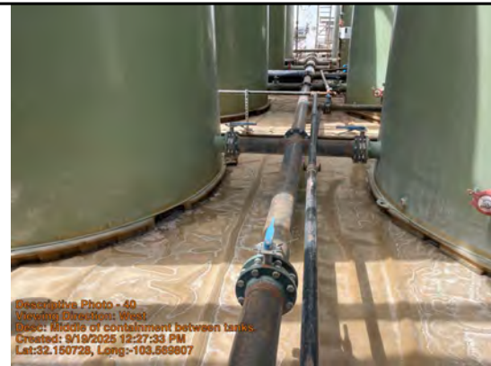
Middle of containment between tanks.
