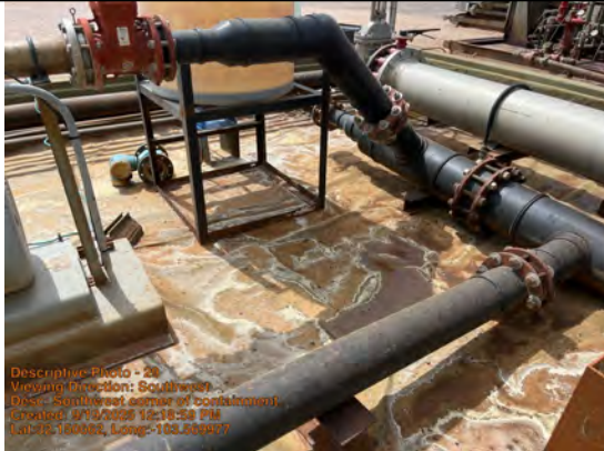
Southwest corner of containment.
