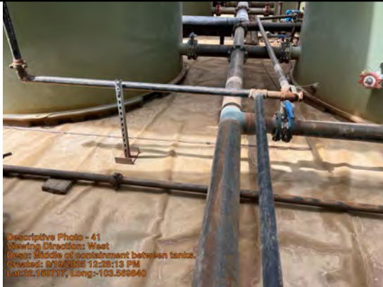
Middle of containment between tanks.
