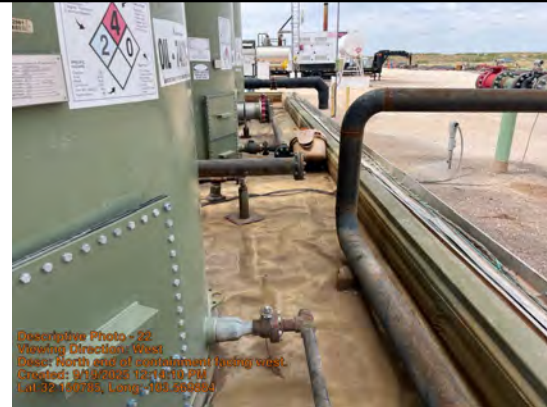
North end of containment facing west.
