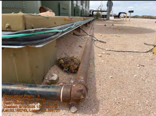
North exterior wall facing west.
