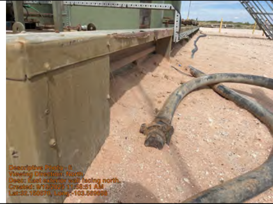
East exterior wall facing north.
