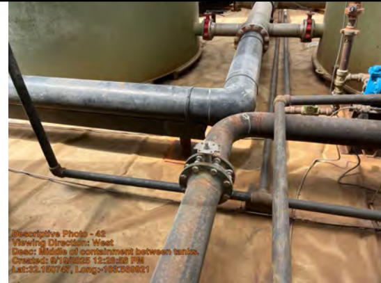
Middle of containment between tanks.
