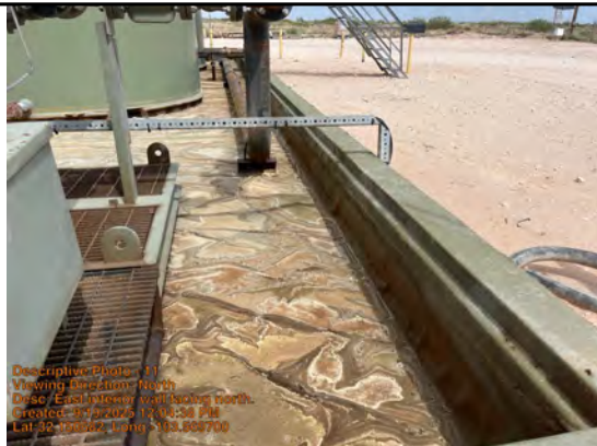
East interior wall facing north.
