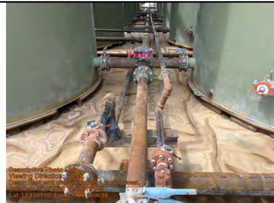
East end of containment facing west.
