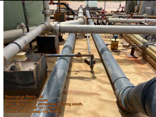
West end of containment facing south.
