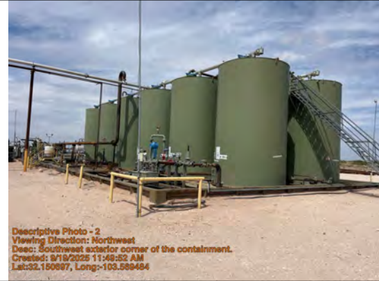
Southeast exterior corner of the CTB.
