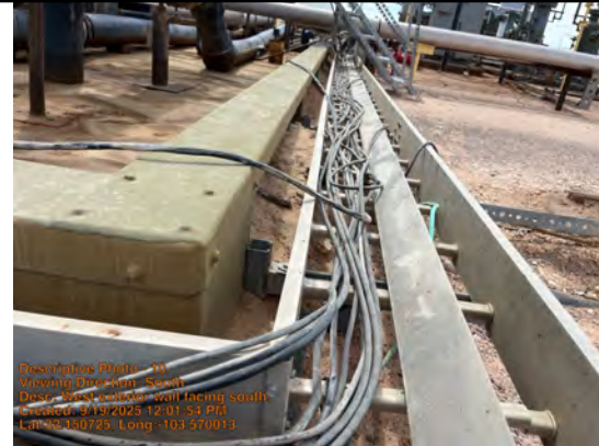
West exterior wall facing south.
