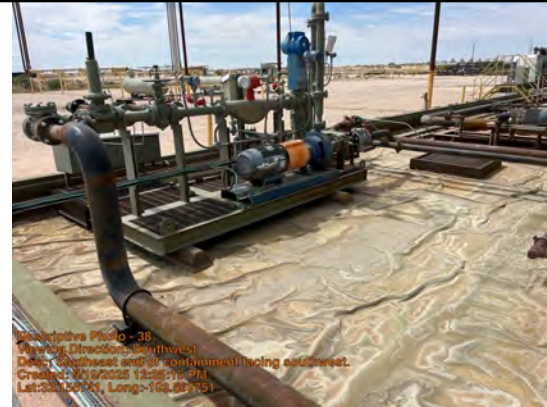
Southeast end of containment facing southwest.
