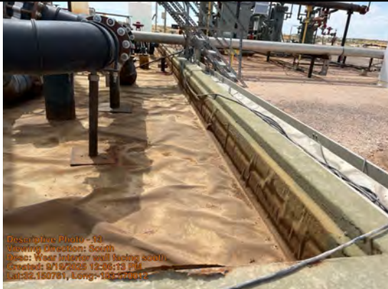
West interior wall facing south.
