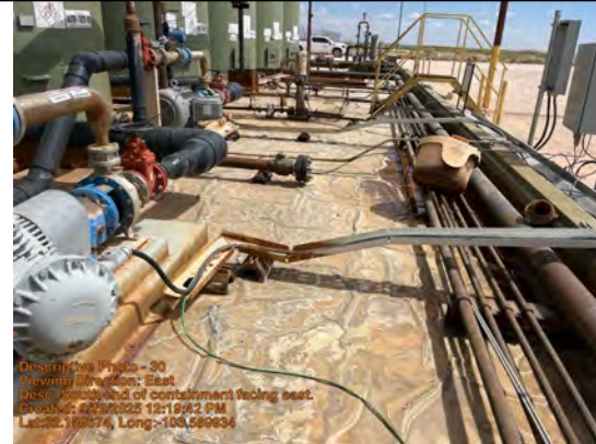
South end of containment facing east.
