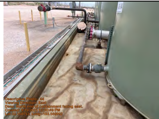
North end of containment facing east.
