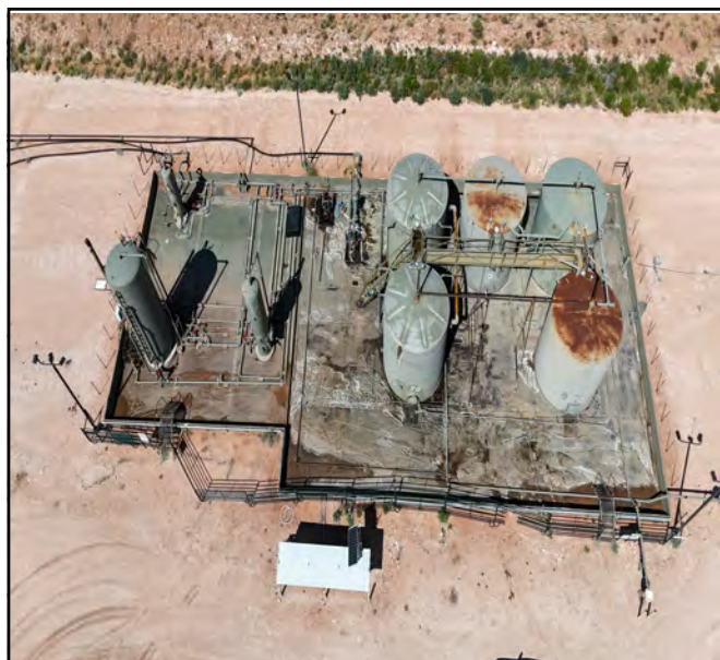
Pre Powerwash aerial photos.
