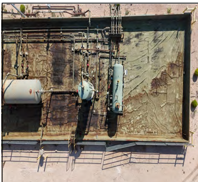
Pre Powerwash aerial photos.
