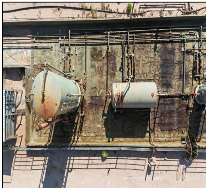
Pre Powerwash aerial photos.
