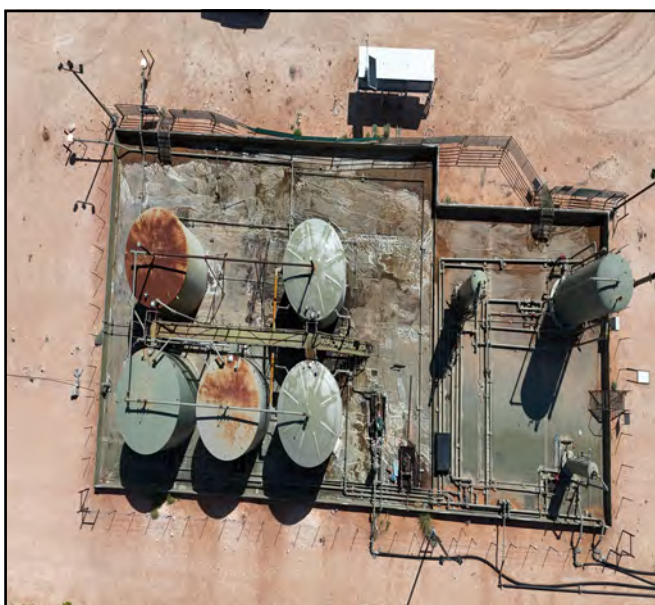
Pre Powerwash aerial photos.
