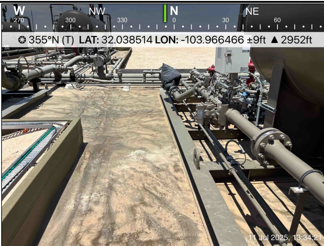
PHOTO 10: Northern view during liner inspection activities. 7/11/2025
