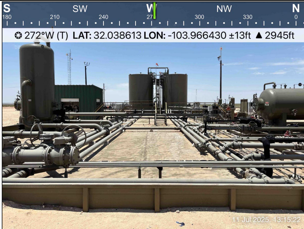
PHOTO 3: Western view outside of containment during liner inspection activities. 7/11/2025
