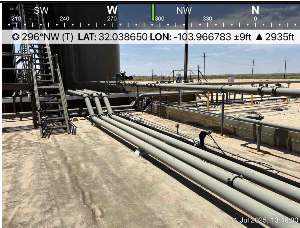
PHOTO 14: Northwestern view during liner inspection activities. 7/11/2025
