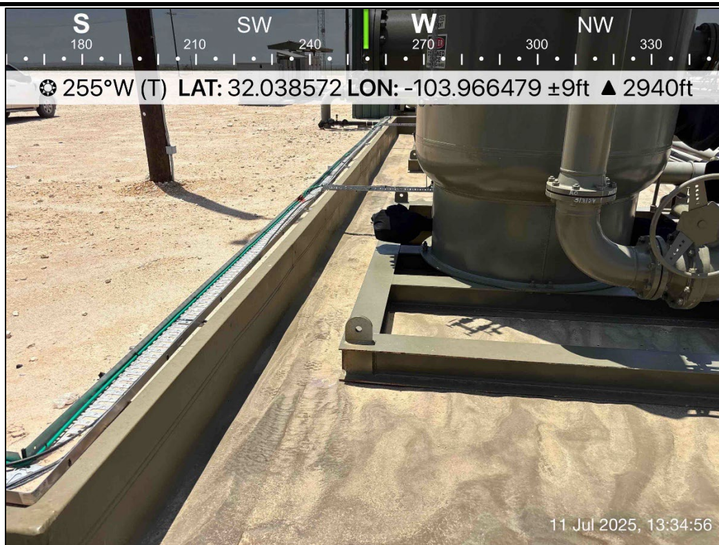
PHOTO 16: Southwestern view during liner inspection activities. 7/11/2025
