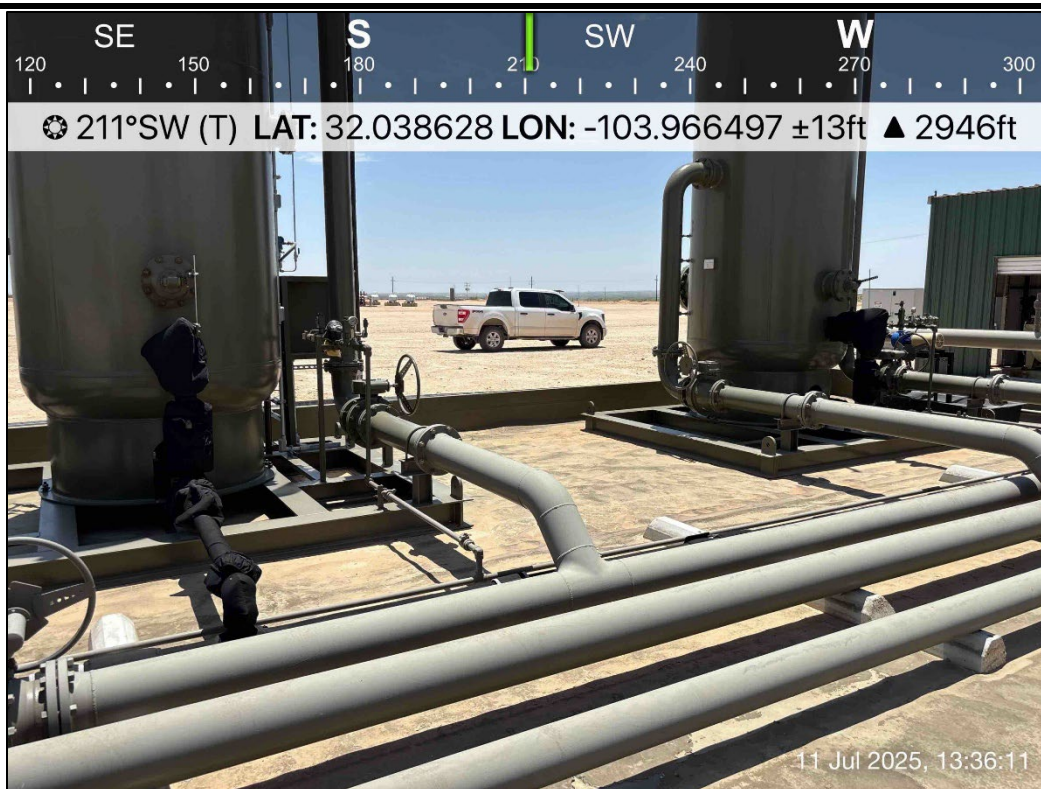
PHOTO 12: Southwestern view during liner inspection activities. 7/11/2025
