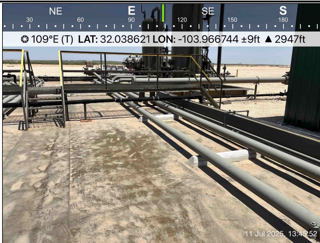
PHOTO 15: Southeastern view during liner inspection activities. 7/11/2025
