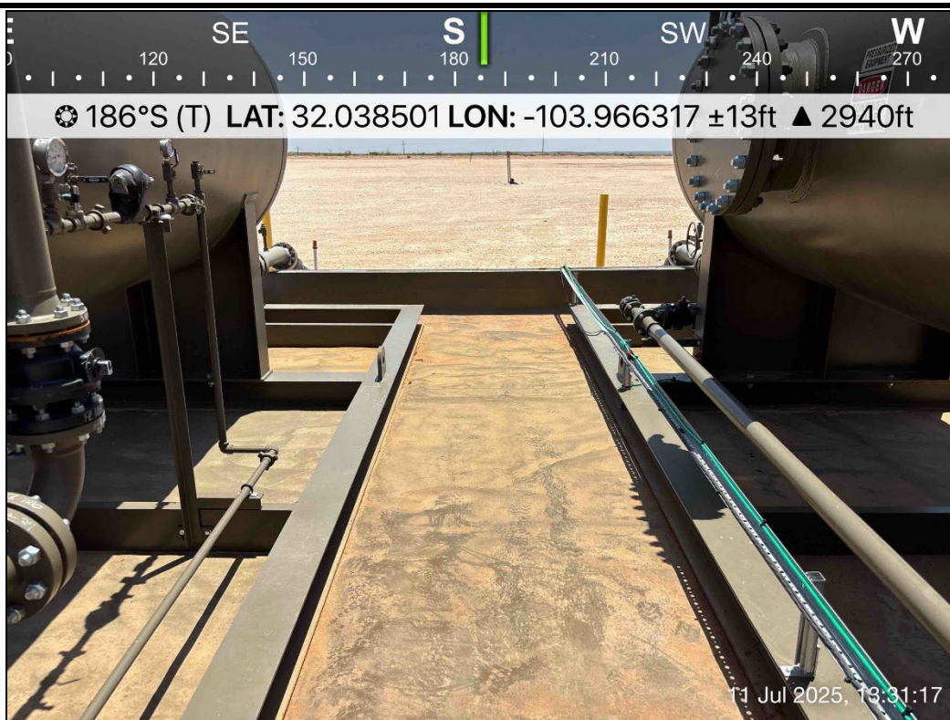
PHOTO 20: Southern view during liner inspection activities. 7/11/2025
