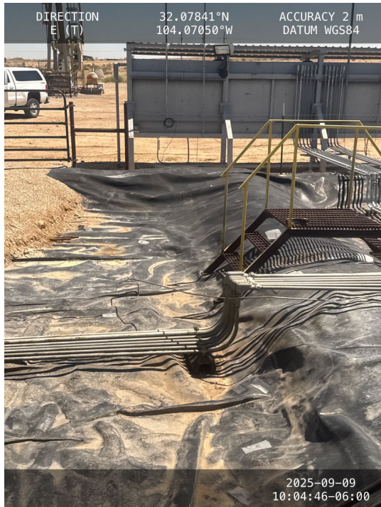
Photo 5 View of southern portion of containment facing east.
