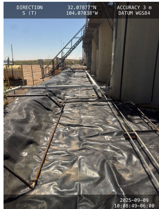
Photo 12 View of eastern portion of containment facing south.
