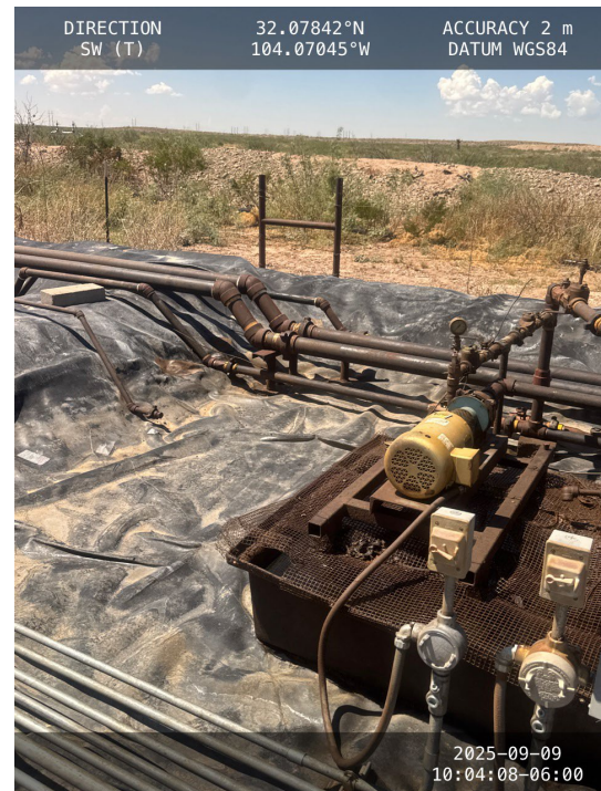
Photo 2 View of Southwest corner of containment facing southwest.
