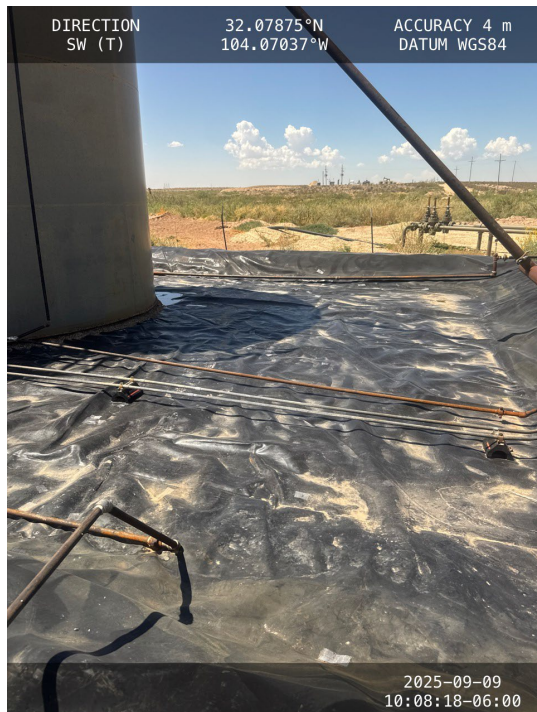
Photo 11 View of northern portion of containment facing southwest.
