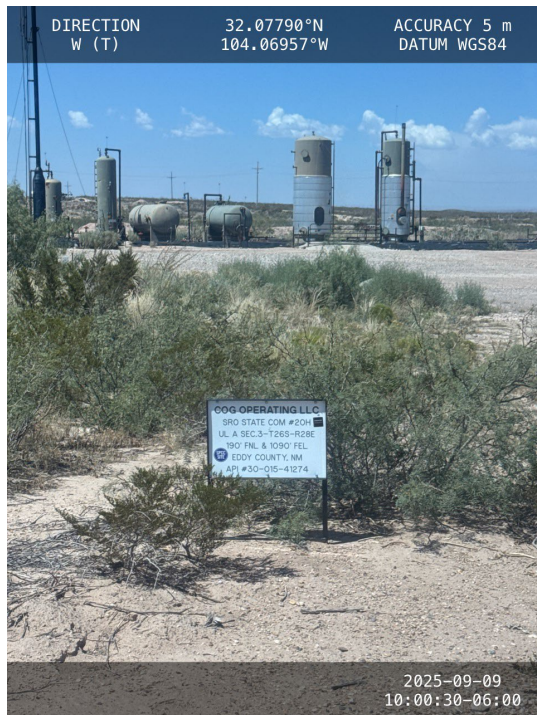
Photo 1 View of Site location.
