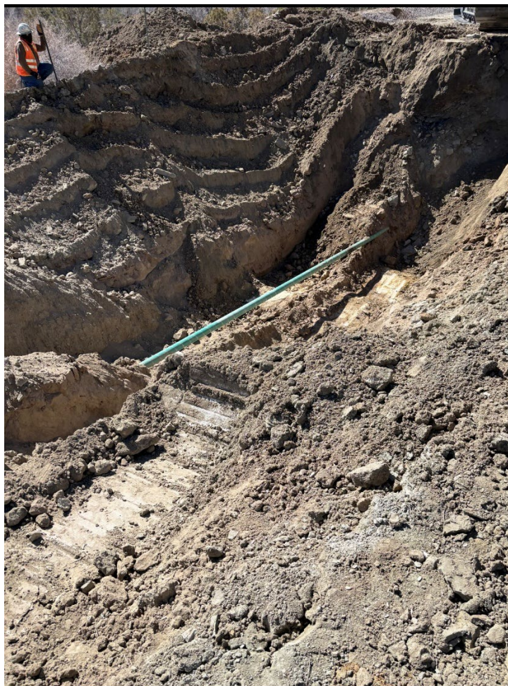
Picture 1: View of Excavation
