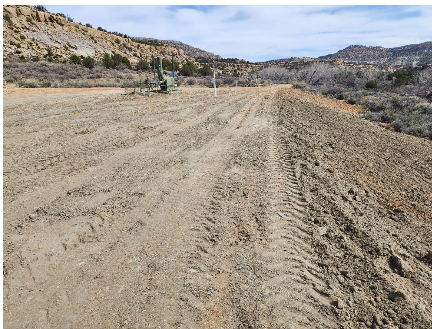
Picture 3: The Scott 13R Excavation Backfilled
