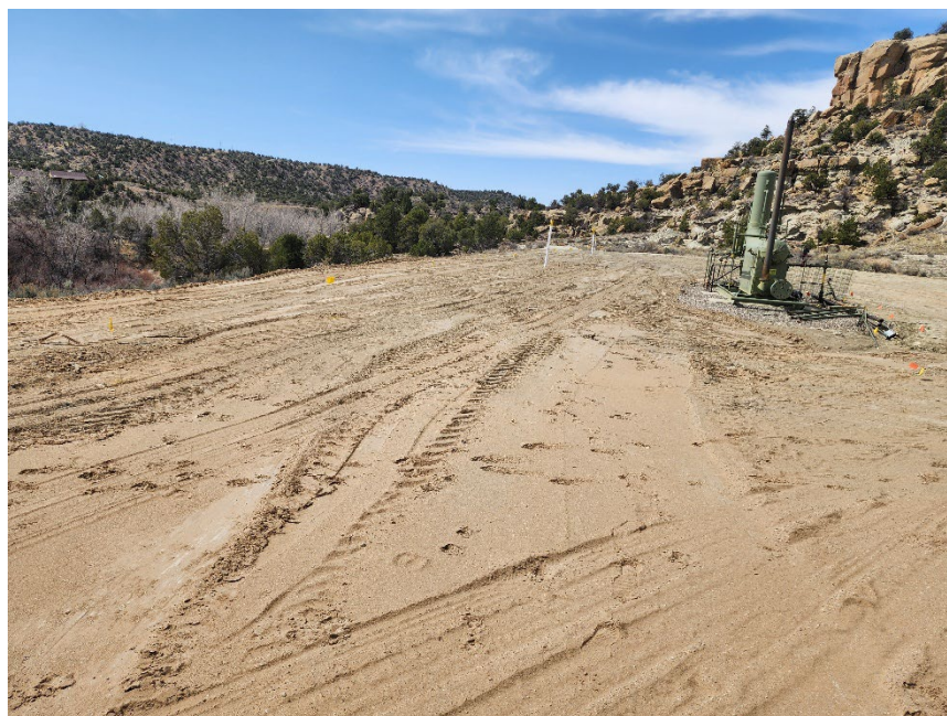
Picture 2: The Scott 13R Excavation Backfilled
