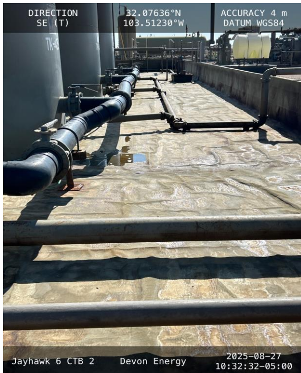
Photo 3 View of southern portion of secondary containment facing southeast.
