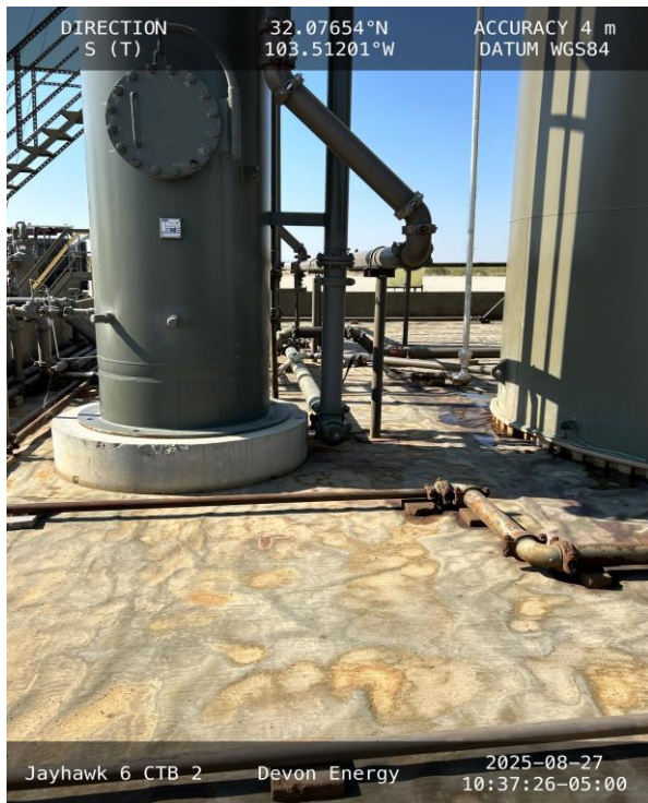
Photo 5 View of eastern portion of secondary containment towards south.
