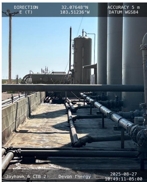
Photo 9 View of northern portion of secondary containment facing east.
