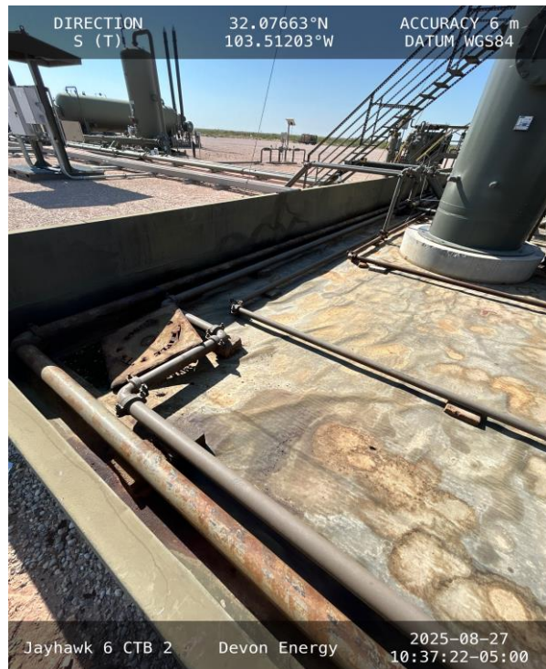
Photo 4 View of northeast corner of secondary containment.
