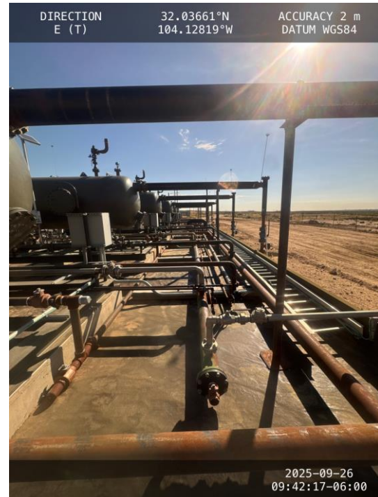
Photo 10 View of containment facing east.
