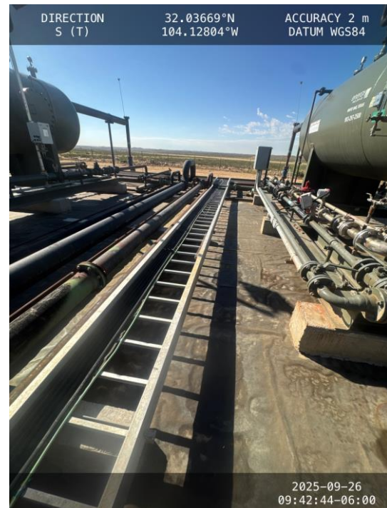
Photo 12 View of central portion of containment facing south.
