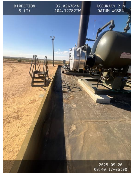
Photo 2 View of containment facing south.
