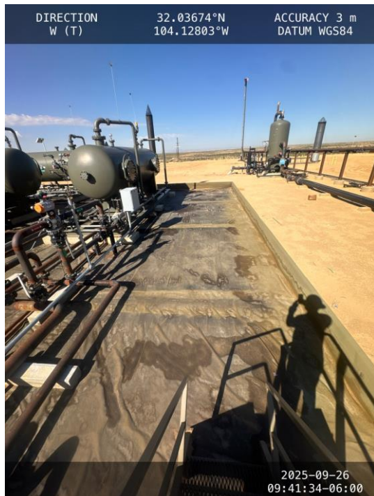
Photo 7 View of containment facing west.
