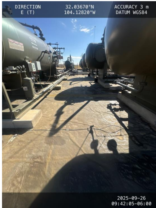
Photo 9 View of central portion of containment facing east.
