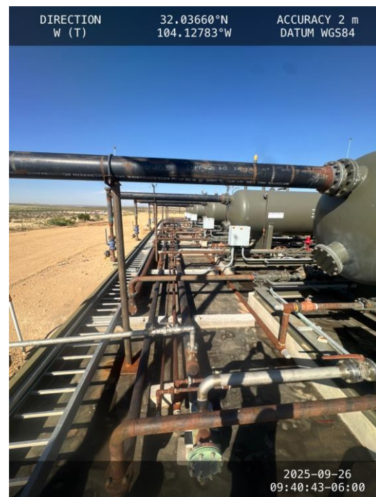
Photo 4 View of containment facing west.
