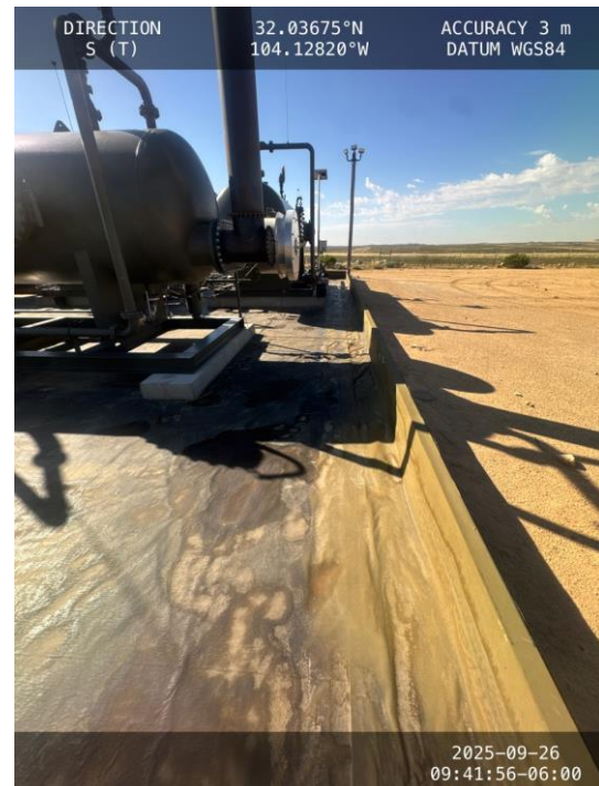
Photo 8 View of containment facing south.
