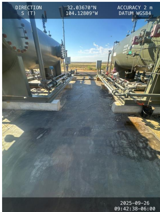
Photo 11 View of central portion of containment facing south.
