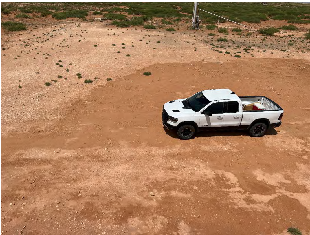
SP-2 – The spill does not cover the entire pad
