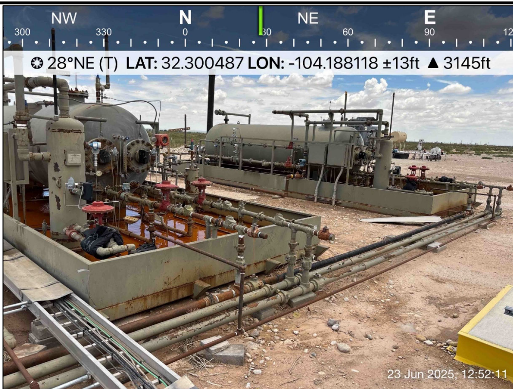
PHOTO 2: Northeastern view during initial site assessment activities. 6/23/2025
