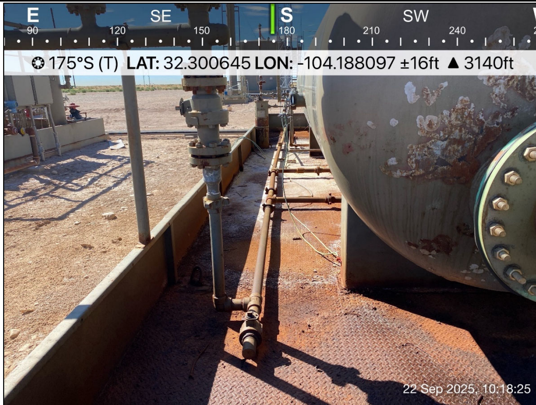
PHOTO 15: Southern view during liner inspection activities. 9/22/2025
