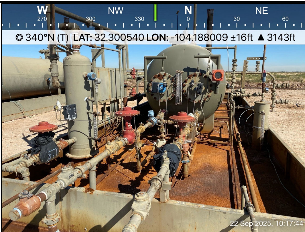
PHOTO 10: Northwestern view during liner inspection activities. 9/22/2025
