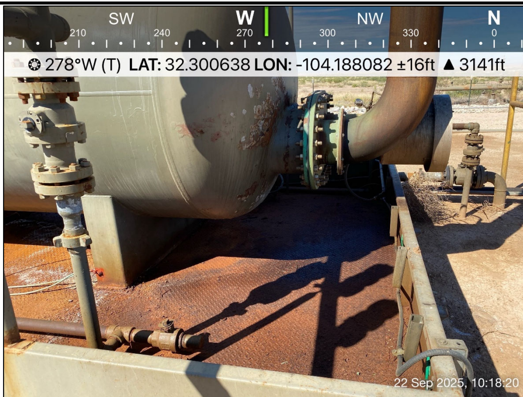
PHOTO 12: Western view during liner inspection activities. 9/22/2025
