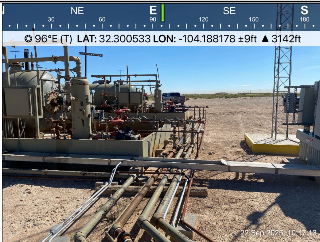
PHOTO 8: Eastern view outside of containment during liner inspection activities. 9/22/2025
