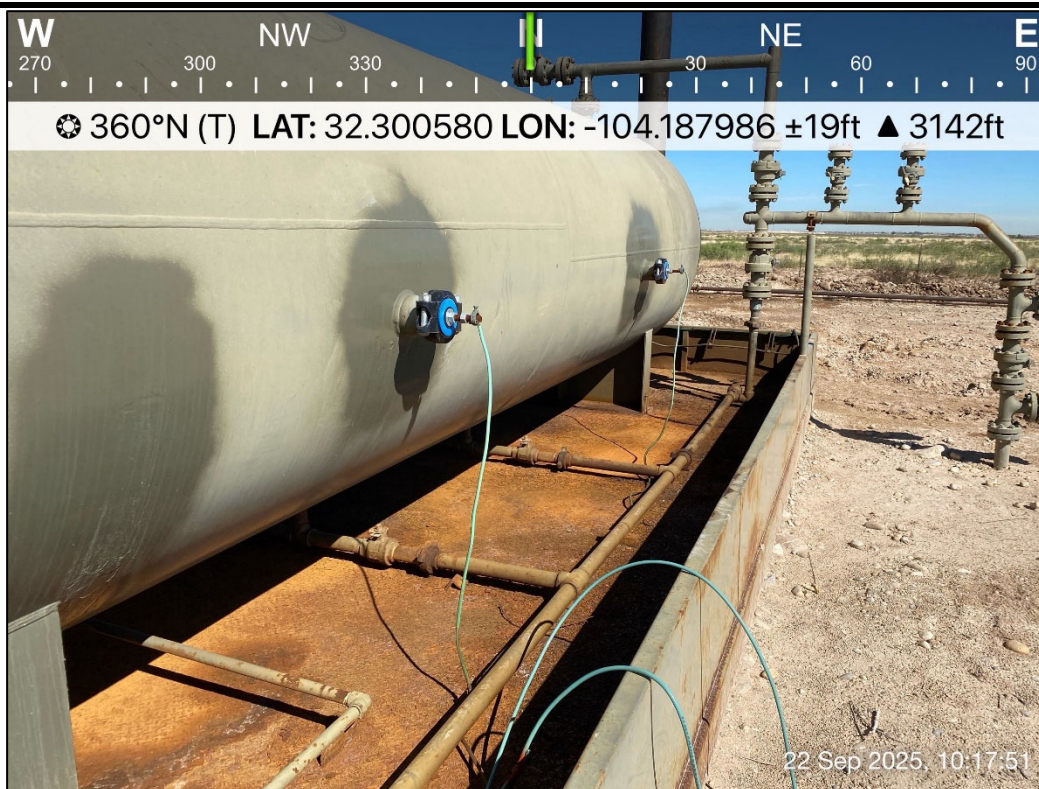
PHOTO 11: Northern view during liner inspection activities. 9/22/2025
