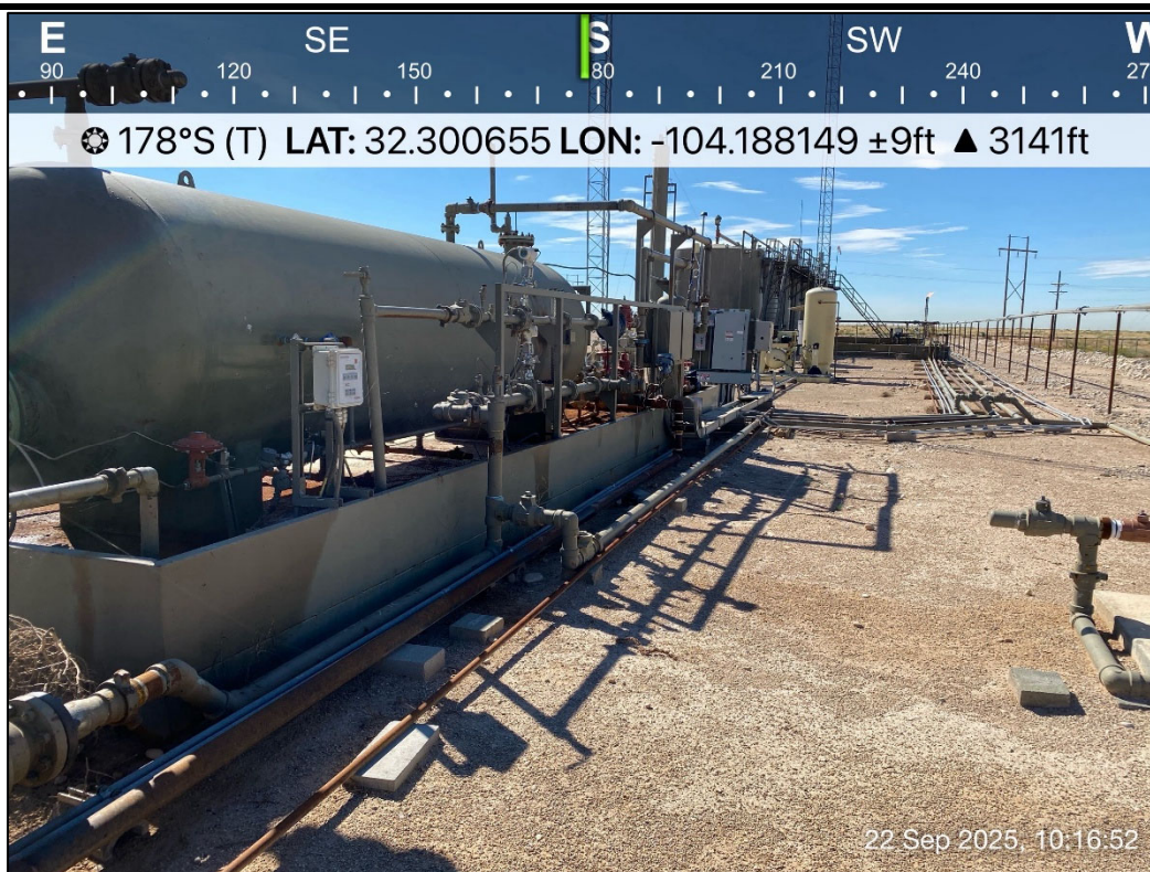
PHOTO 7: Southern view outside of containment during liner inspection activities. 9/22/2025
