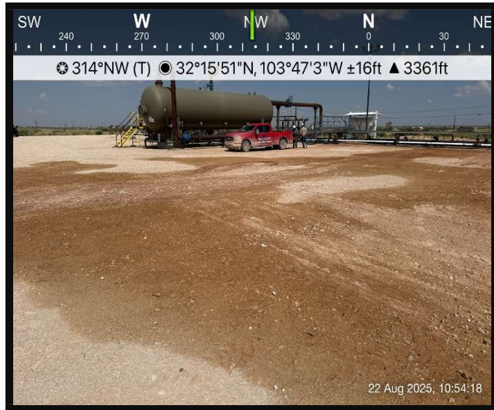
View of Area of Concern
