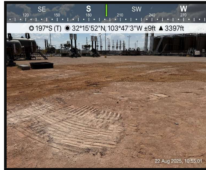
View of Area of Concern
