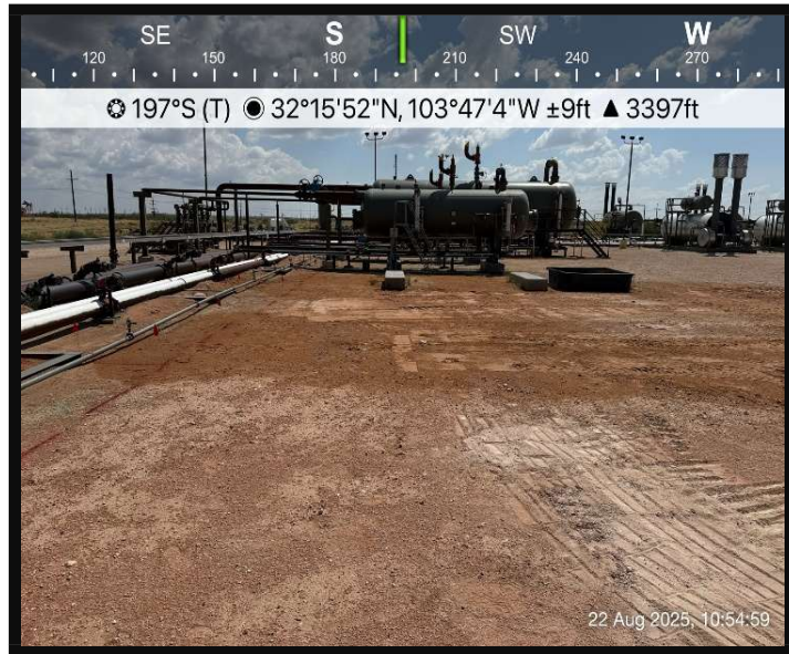
View of Area of Concern
