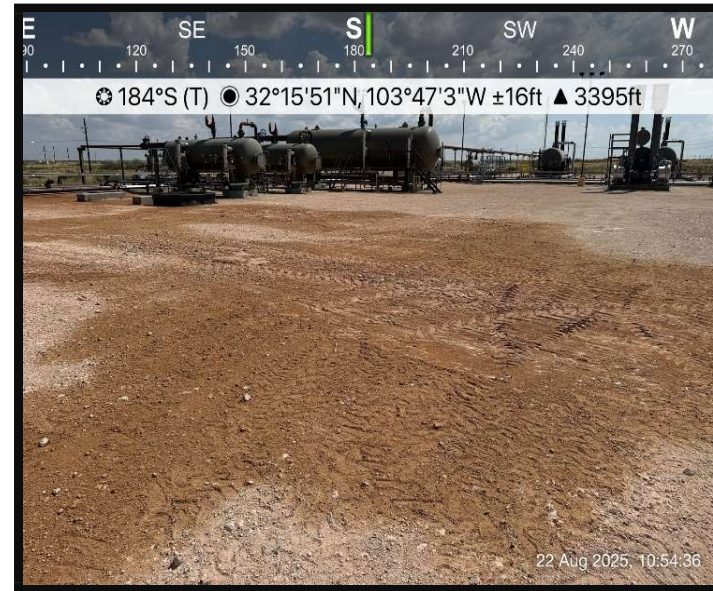
View of Area of Concern
