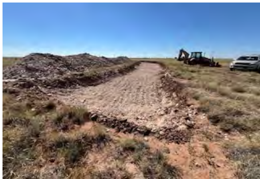
View to S of excavation.
