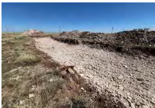
View to N of excavation.
