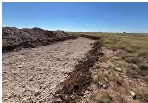
View to S of excavation.
