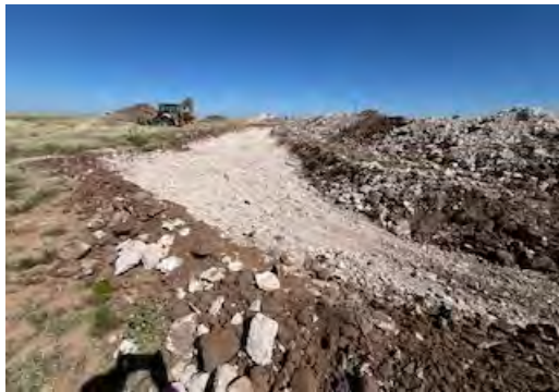
View to N of excavation.
