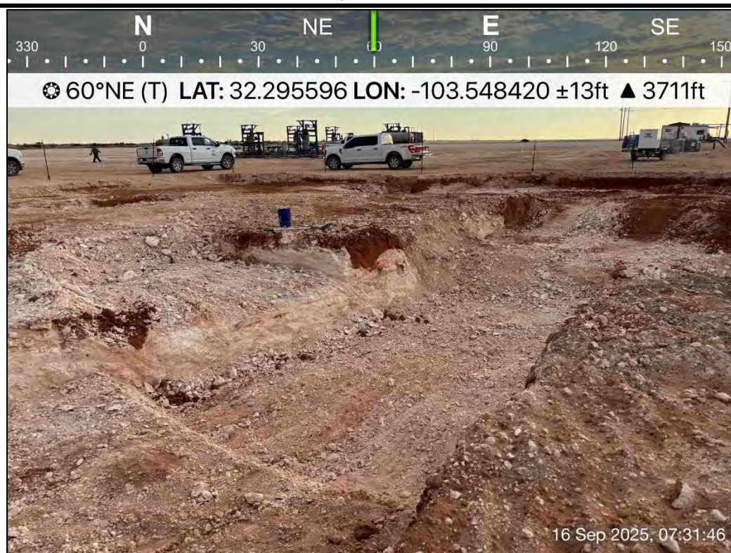
PHOTO 12: Northeastern view of excavation extent following additional excavation activities. 9/16/2025
