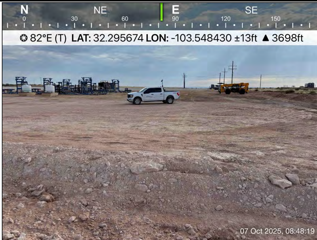
PHOTO 15: Eastern view following restoration activities. 10/7/2025
