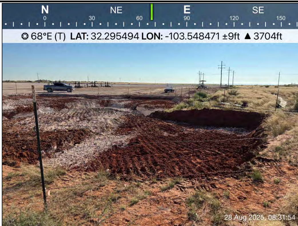
PHOTO 9: Northeastern view of excavation extent. 8/28/2025
