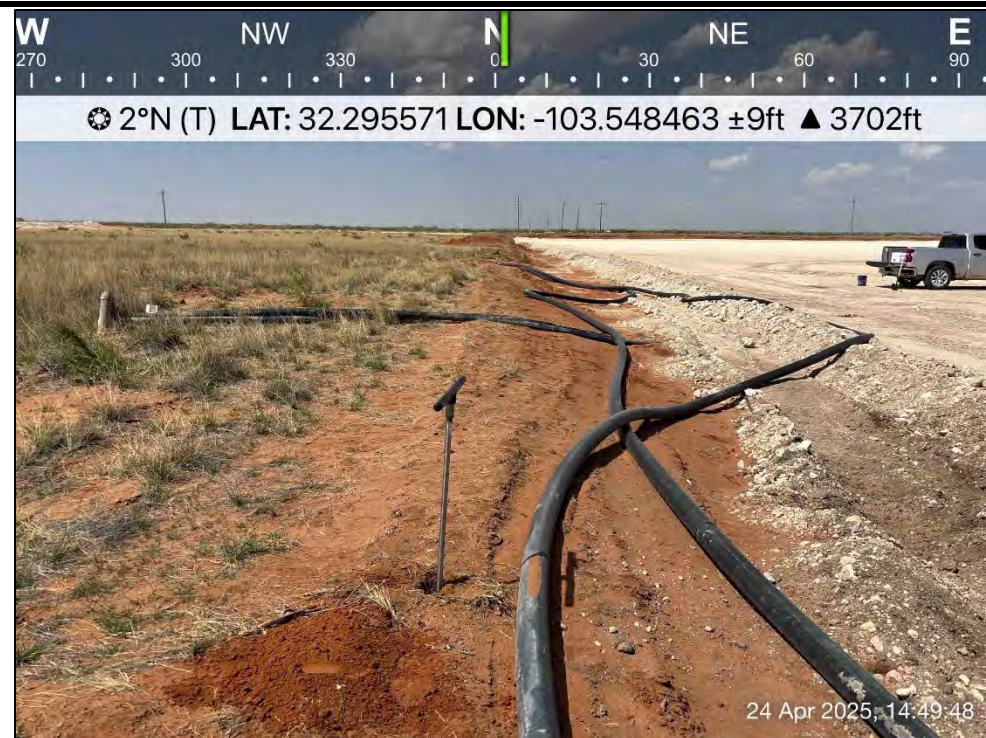
PHOTO 6: Northern view during initial delineation activities. 4/24/2025
