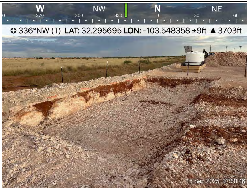
PHOTO 11: Northwestern view of excavation extent following additional excavation activities. 9/16/2025
