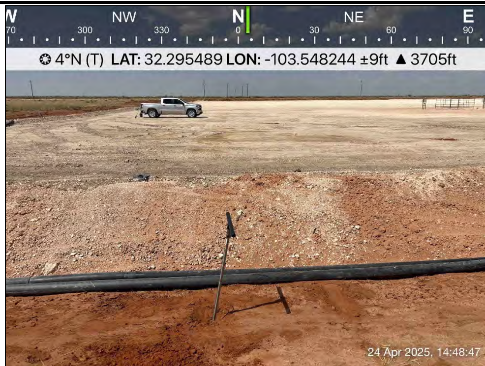
PHOTO 5: Northern view during initial delineation activities. 4/24/2025
