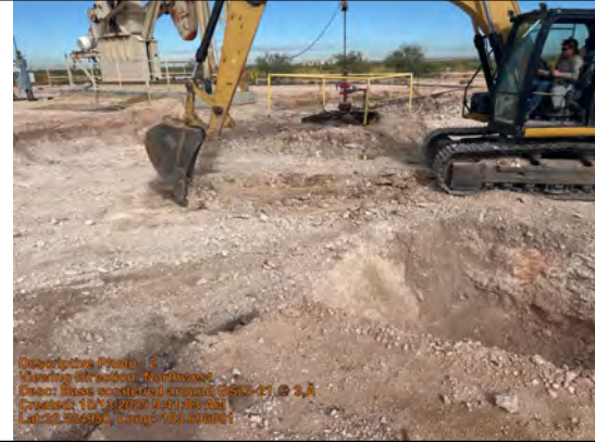
Excavation around BS25-21 @ 3'
