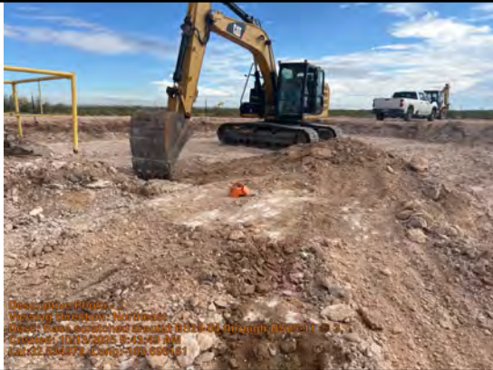
Excavation around BS25-04 through BS25-11 @ 3'
