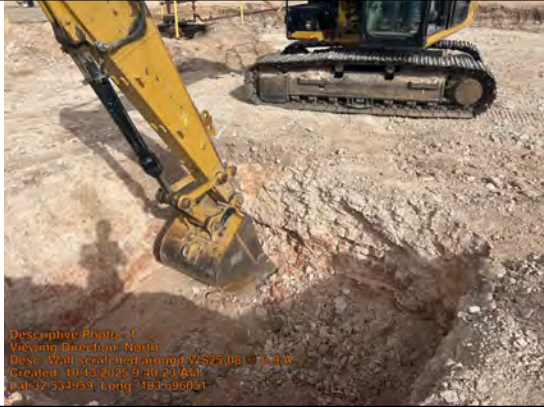
Excavation around WS25-08 @ 0-9'
