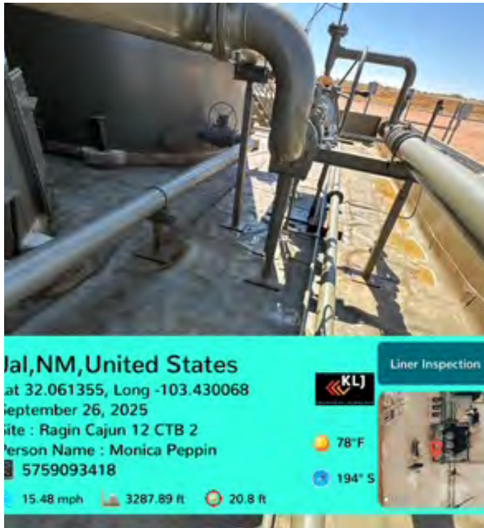
West side of containment facing south from near middle tank.
