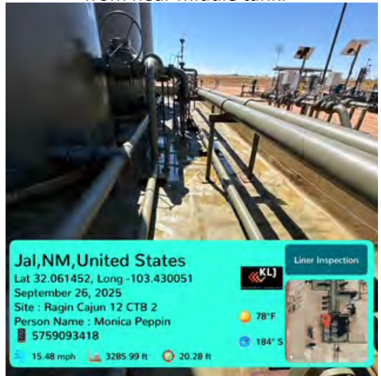
West wall facing south from north end.
