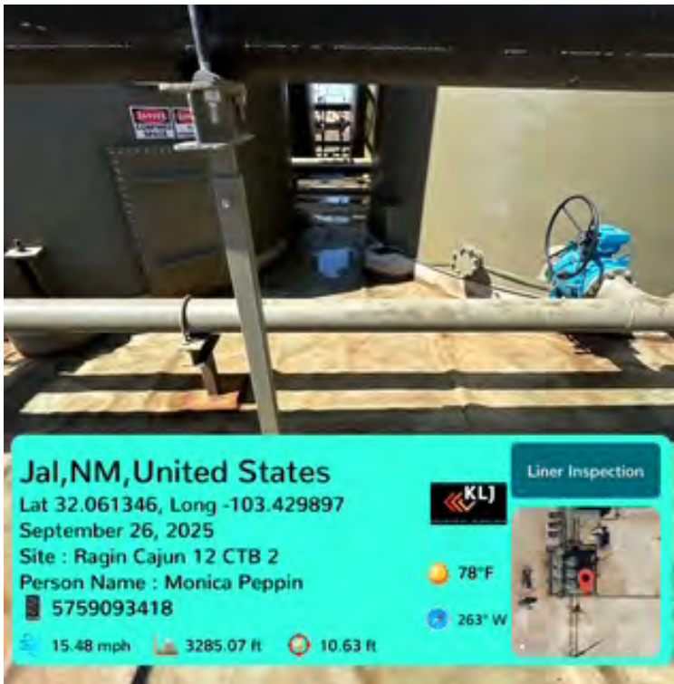
Liner between middle tanks from east side facing west.
