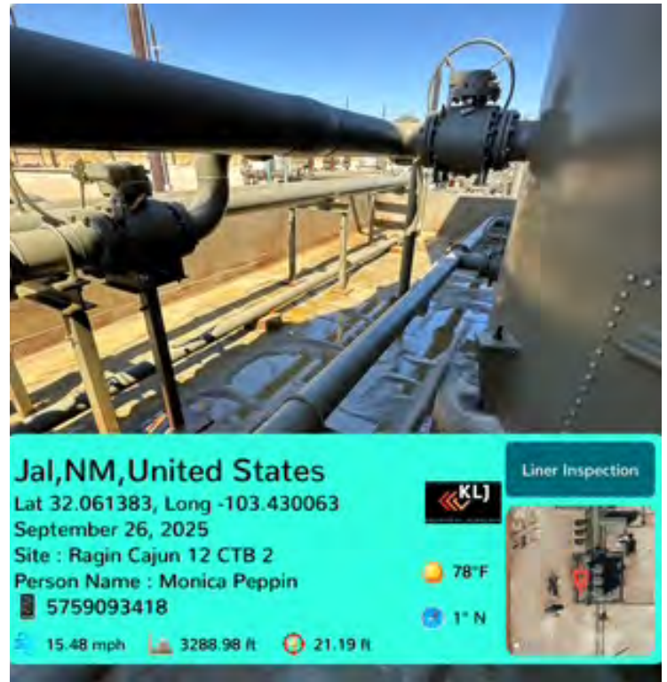
Facing north viewing liner on west side from near middle tank.
