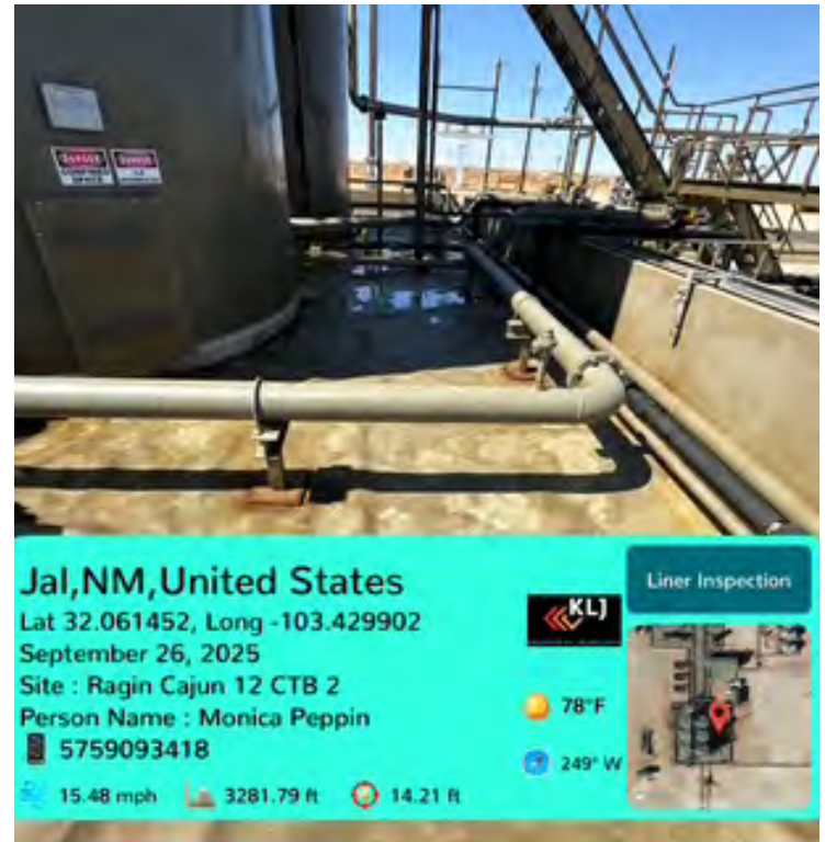
North area of containment facing west from northeast corner.
