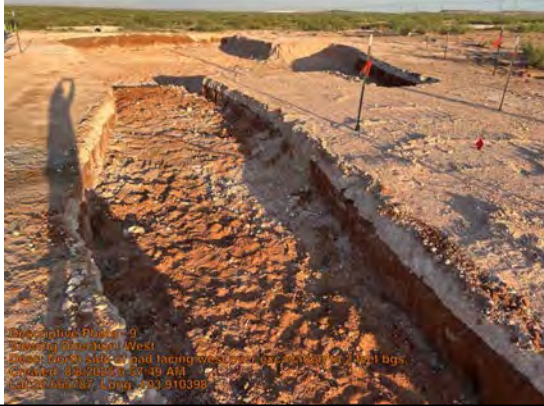
Viewing Direction: West
