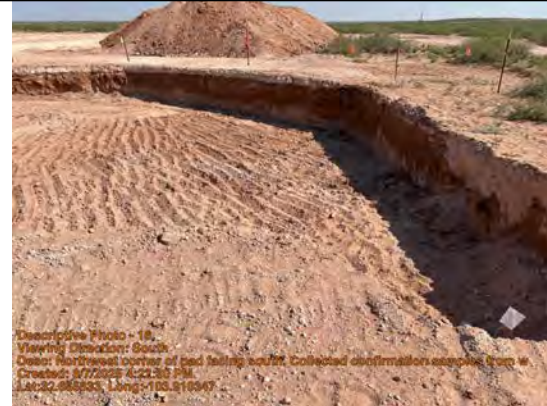
Viewing Direction: South
