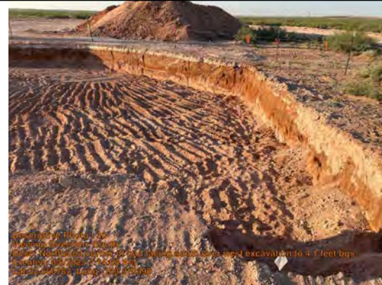
Viewing Direction: South
