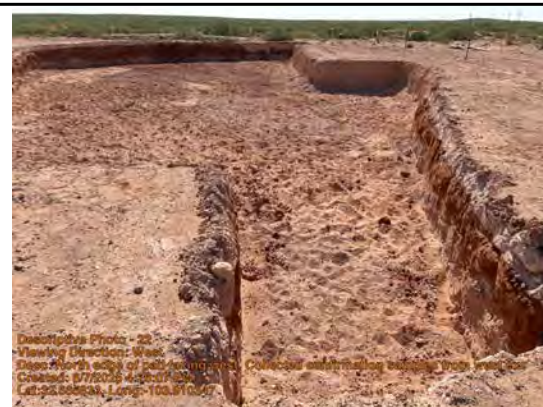
Viewing Direction: West
