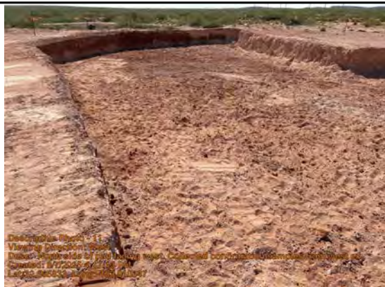
Viewing Direction: West
