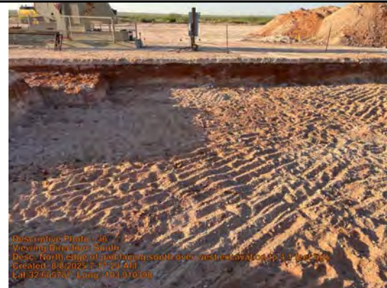
Viewing Direction: South
