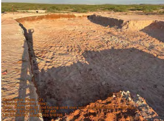
Viewing Direction: West
