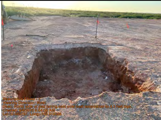
Viewing Direction: West
