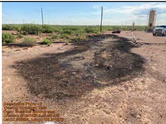
West toe looking east
