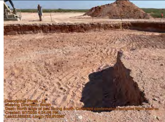
Viewing Direction: South
