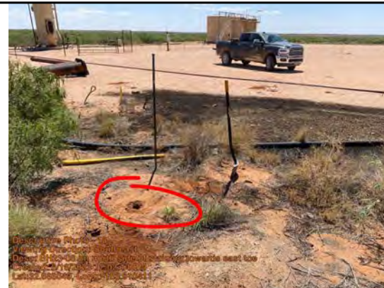
BH23-08 on north side of staining towards east toe
