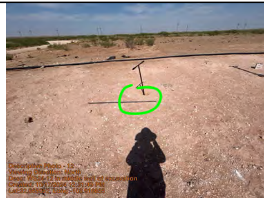
WS24-12 in middle wall of excavation
