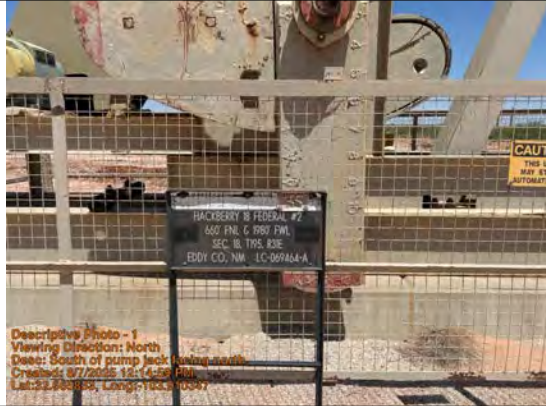
South of pump jack facing north.
