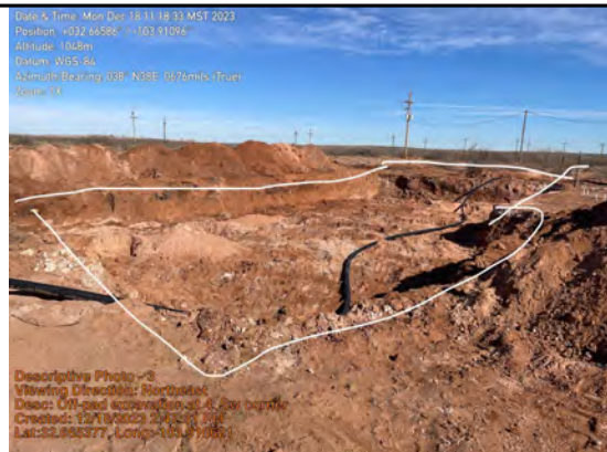
West excavation at 4. Sw corner
