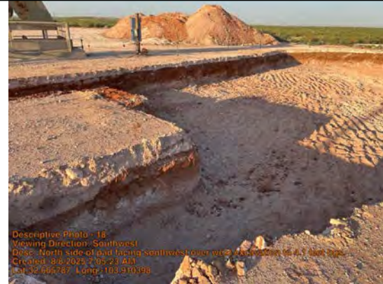
Viewing Direction: Southwest
