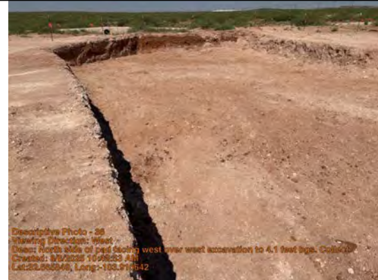
Viewing Direction: West
