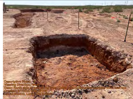
North side of pad facing west. Collected confirmation samples from east excavation to 4.1 feet bgs.
