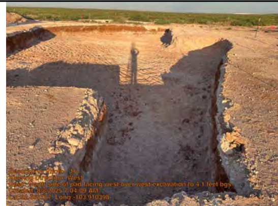
Viewing Direction: West
