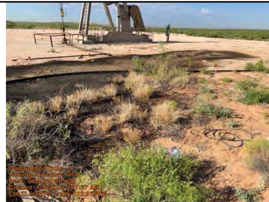
Staining off pad
