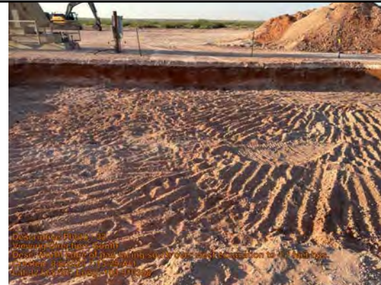
Viewing Direction: South
