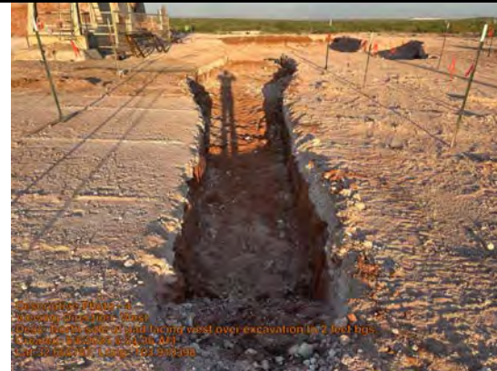
Viewing Direction: West
