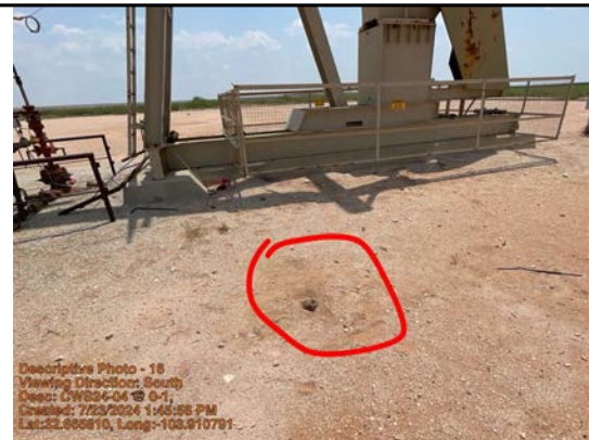
Viewing Direction: South
