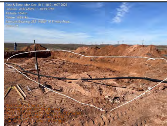
West excavation at 4. SE corner
