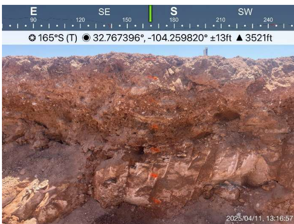
Figure 18. Excavation Depth verification.
