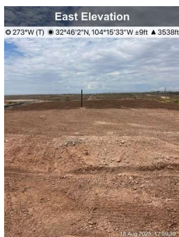
Figure 23. Excavation backfilled and seeded.
