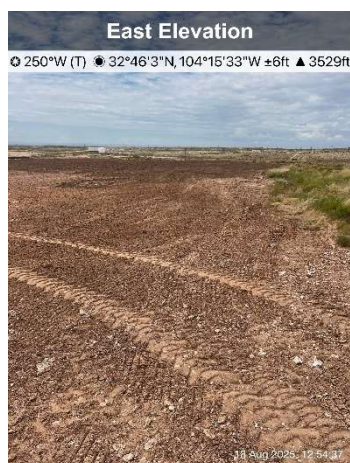
Figure 21. Excavation backfilled and seeded.
