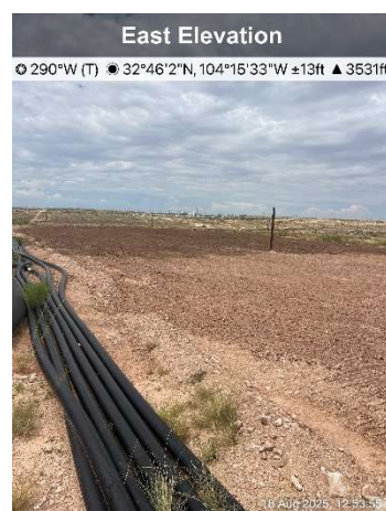
Figure 24. Excavation backfilled and seeded.
