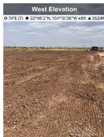
Figure 22. Excavation backfilled and seeded.
